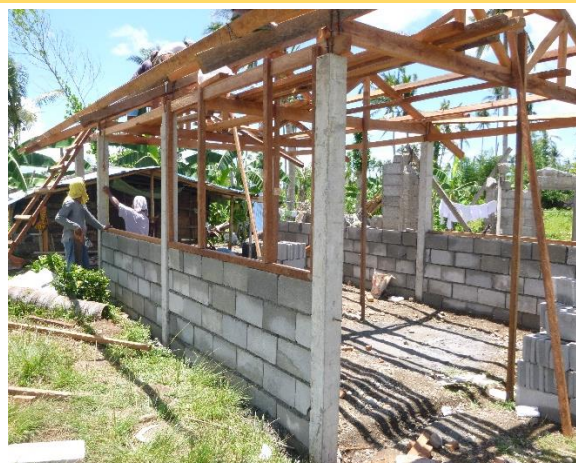
Figure 1: Concrete blocks have been installed between the reinforced concrete columns, up to the level of the window sill of this core shelter in Tabontabon, Leyte. Credit: Philippines Red Cross Haiyan Shelter Programme (Photo W. Eastwood)
