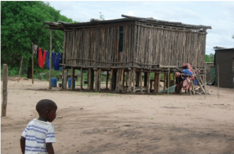
An example of an elevated house in Chicualacuala
