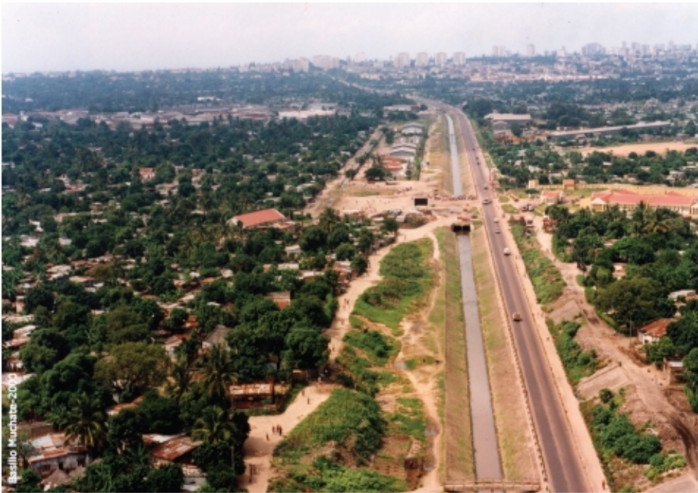
Maputo, the main drainage
