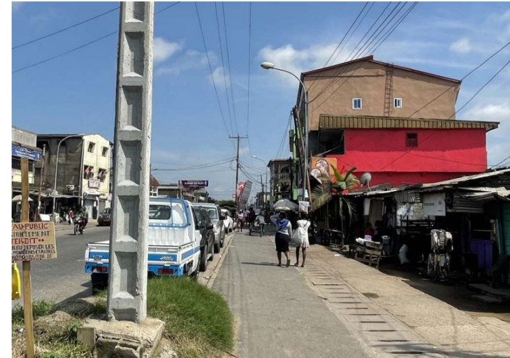
Photo 5. Buildings in official lands along the asphalted road Source: UN-Habitat
