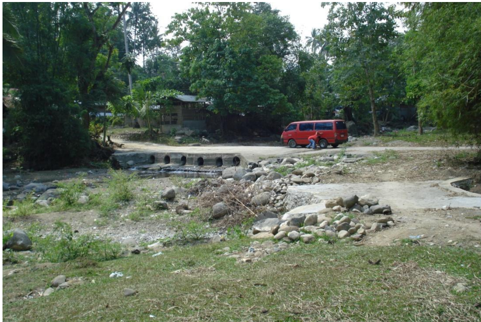
Photo 2. Flooding along Malindawag Creek affects nearby Zone 4 in Brgy. Abuno.
