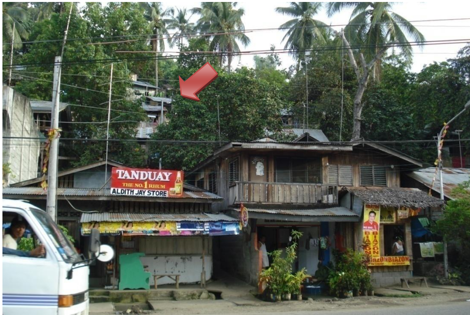
Photo 6. Numerous houses (indicated by red arrow) were built on steep slopes along the highway in Purok 1B, Brgy. Buruun.
