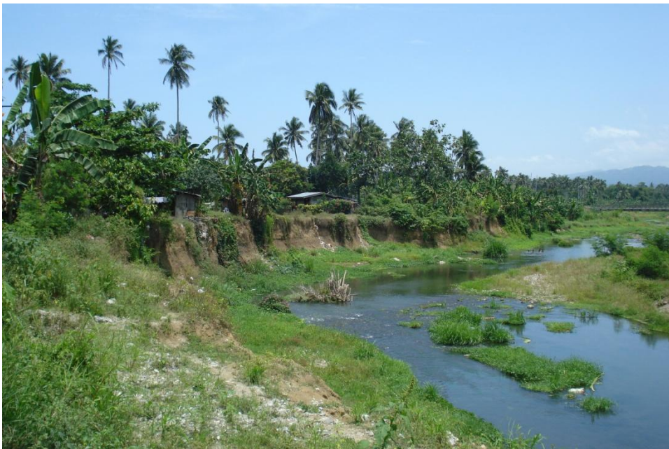
Photo 16. Extensive scouring along this stretch of Iligan River in Purok La Purisima, Baraas, Brgy. Tubod destroyed several houses along the river.
