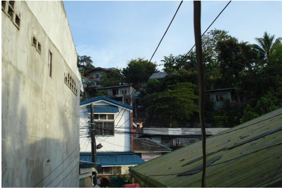
Photo 9. Houses built on steep slopes such as these in Purok 17 Hilltop in Brgy. Tomas Cabili are high risk in terms of landslide.
