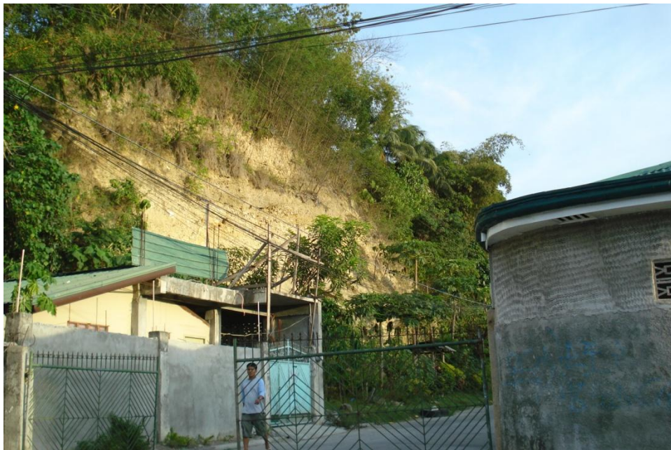
Photo 10. Houses proximal to this limestone cliff in Masinag Subdivision, Purok 15A in Brgy. Tomas Cabili are high risk in terms of landslide.
