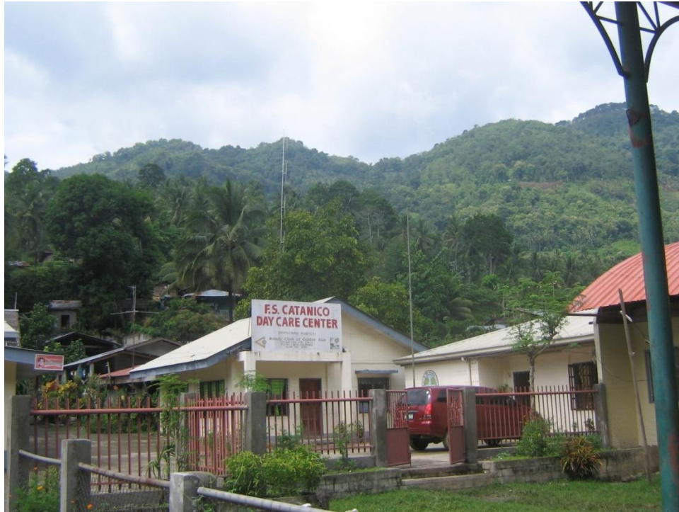
Slopes bounding Brgy. Proper F.S. Catanico with moderate susceptibility to landslides.
