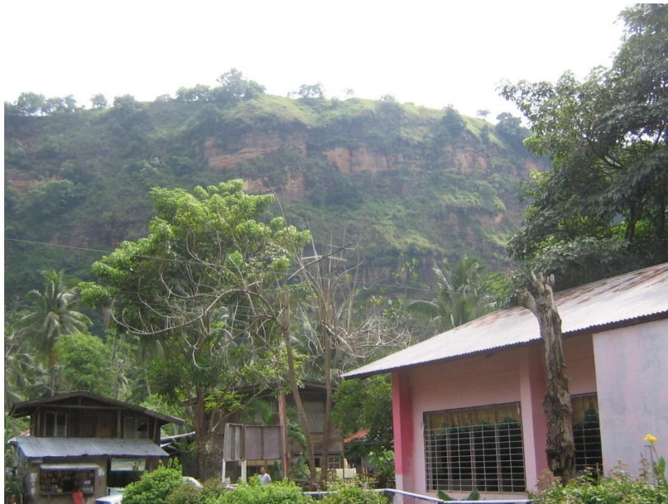
Nearly vertical slopes along Cugman River in Brgy. F.S. Catanico.
