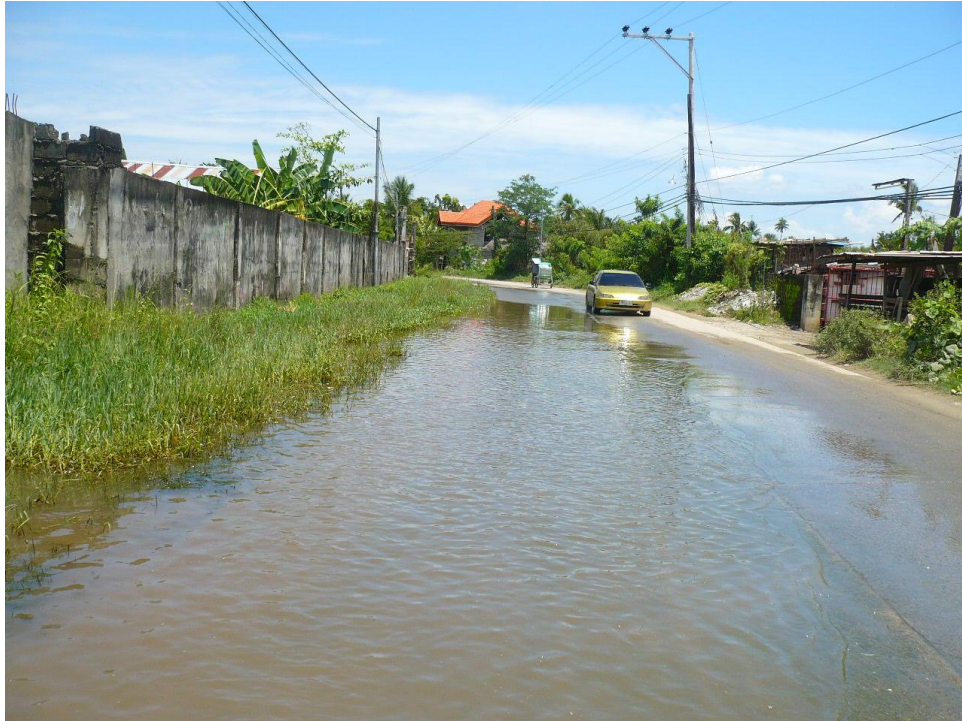
Excessive surface run-off from Brgy. Kauswagan perennially floods Zone 6, Brgy. Bayabas.
