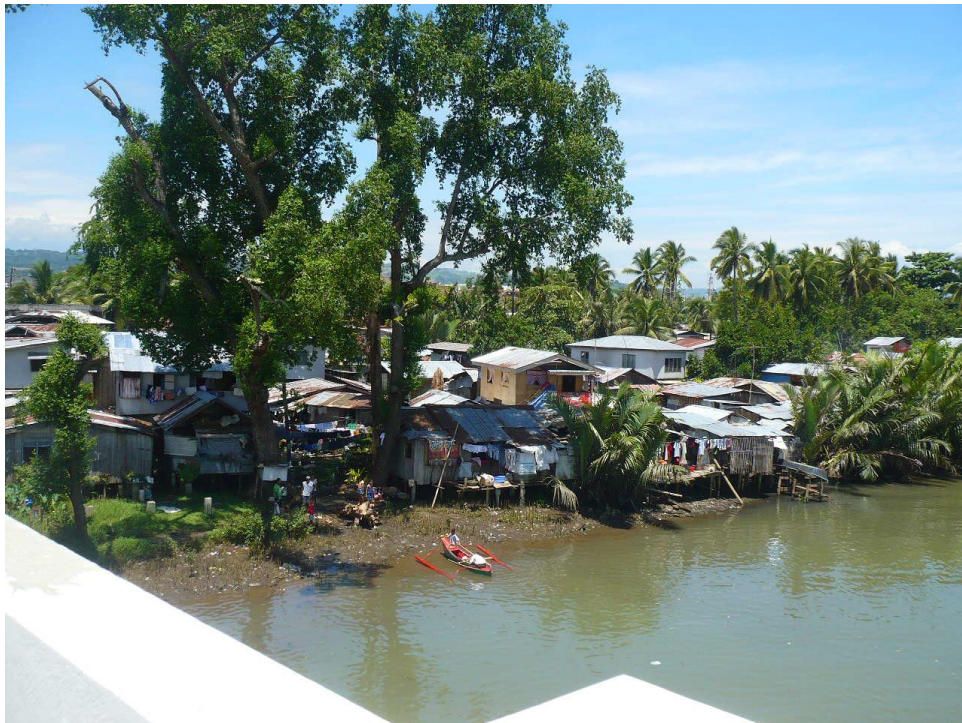
Houses built along the floodplains of Cagayan de Oro River in Brgy. Puntod are highly susceptible to flooding.
