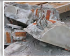
Poor, weak connections between tie columns and bond beams
