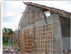
Very tall, slender walls with gable, with overturning failure
