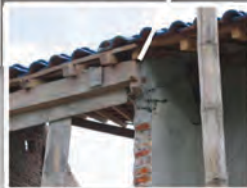
Poor, weak connections between tie columns and bond beams
