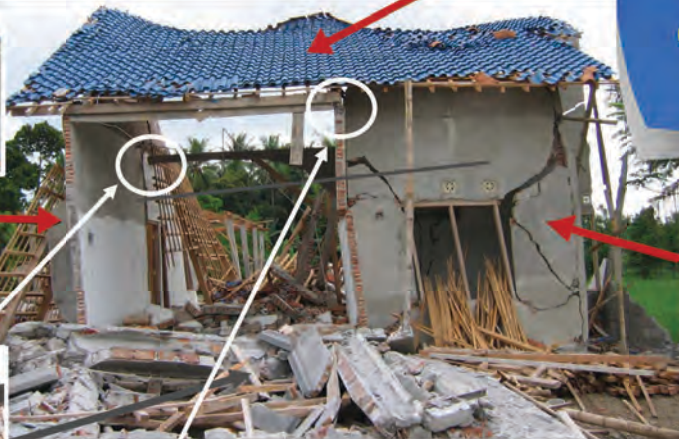
Poor, weak connections between tie columns and bond beams
