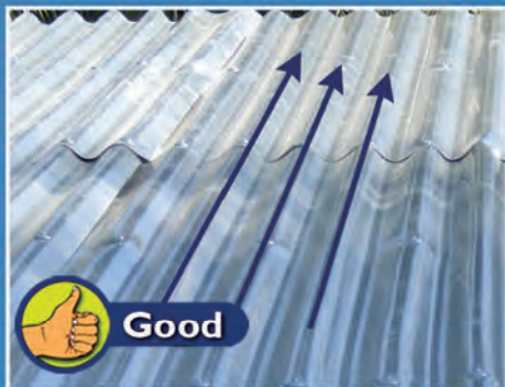
Good connection, waves straight
