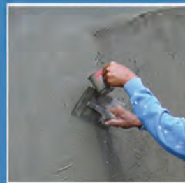
Finish the wall with cement-water slurry
