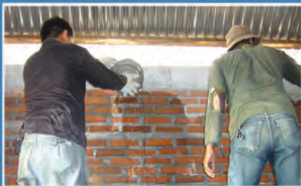
Wet the wall before applying plaster
