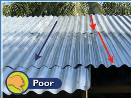
Bad connection, waves not straight
