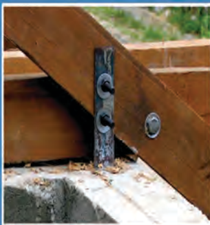
U-shaped plate in the ring beam
