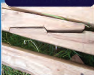
Beam-Beam Splice
