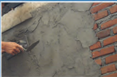
Use pressure to apply the plaster to the wall; do not just throw the plaster against the wall
