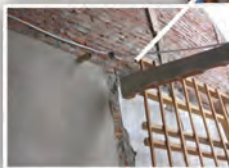
Very tall, slender walls with gable, with overturning failure
