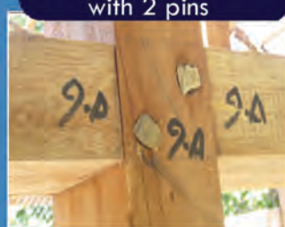
Fasten each joint with 2 pins
