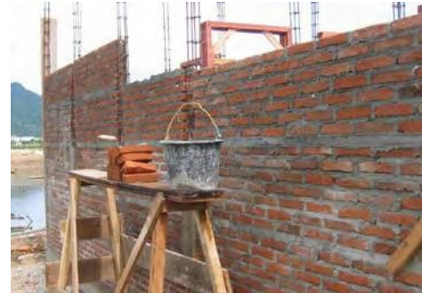
Figure 6. Wall with Horizontal Reinforcement.
