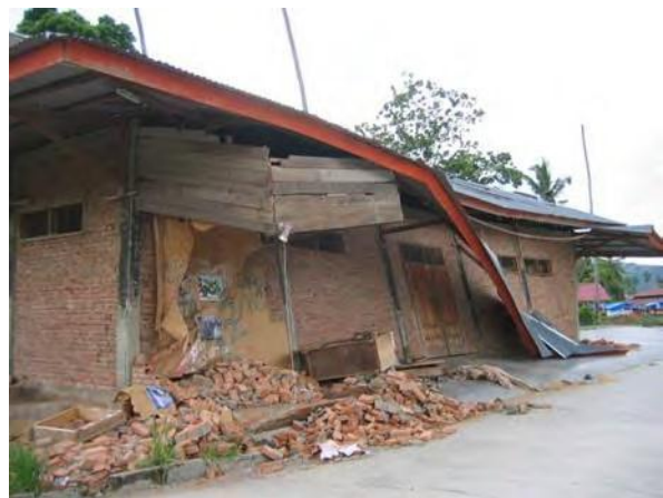
Figure 12. Confined masonry warehouse with overturning failure of long walls without cross-bracing, , IMG 8891
