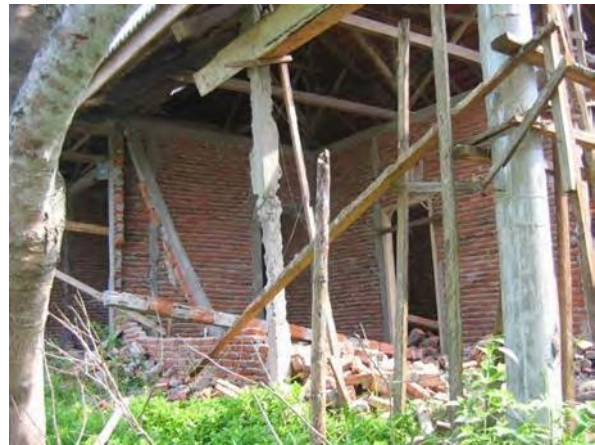
Figure 22. Confined masonry house with failure in masonry walls and connections between tie columns and bond beams, Kec. Airnapal (North Bengkulu)
