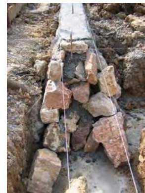
Figure 11. Poorly built stone masonry strip footing. Note gaps between stones, stones standing on end.
