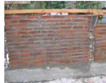
Figure 17. Typical wall built by Build Change-trained mason
