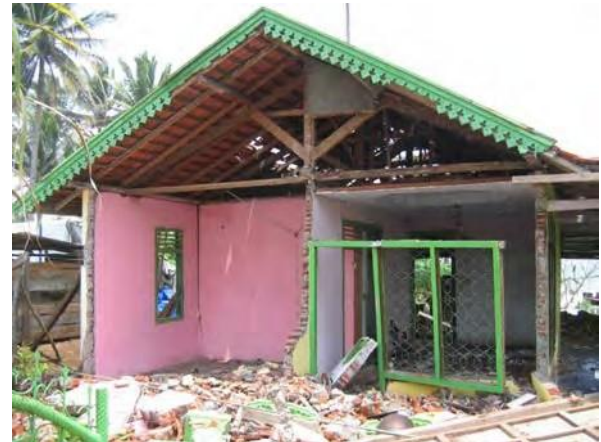
Figure 9. Partially collapsed brick masonry house with RC tie columns and timber bond beams, note partial collapse of masonry gable wall, and lack of in-plane stiffness in front wall, Kec. Lais (North Bengkulu) S3.53217° E102.03771
