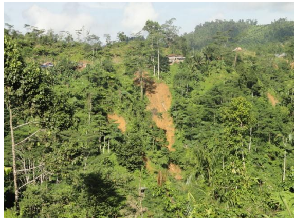
Photo 4. Active landslides near houses in road going to Po. Depot, Brgy. Upper Ulip
