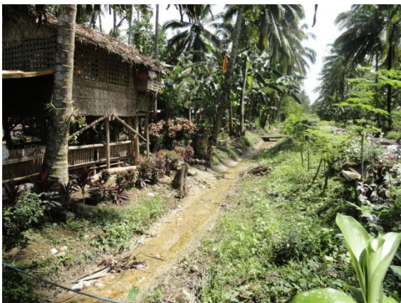
Photo 5. P6, Brgy. Naboc which experience regular flooding due to canal overflows.
