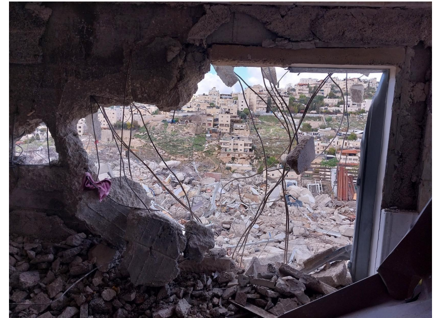
Demolition Incident in Ras Al 'Amud – East Jerusalem
