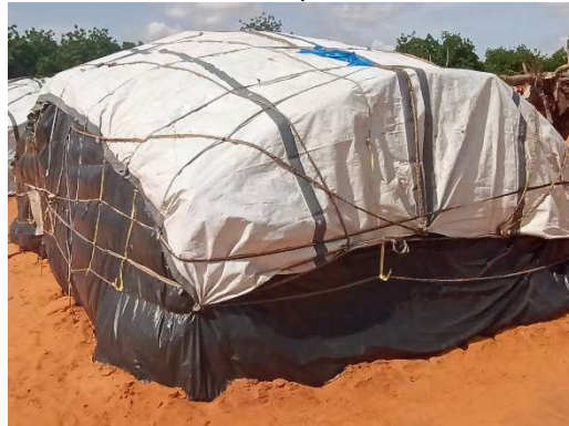
Reinforced shelter with palm doum matt ties
