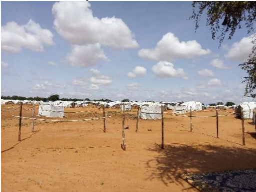
PVC and eucalytus wood, used to build a Mosque
