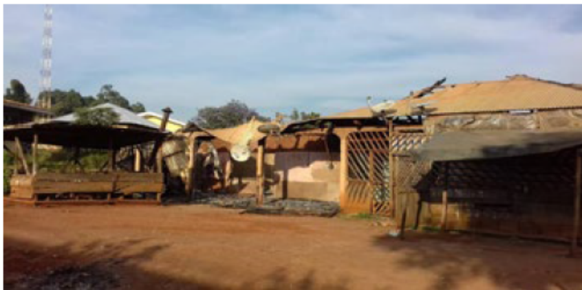
@Global Shelter Cluster Kumbo damages in semi-urban area 2018
