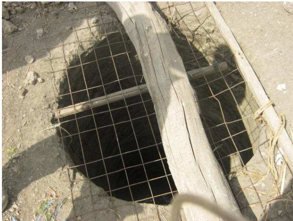
Image 7: An example of a 4m deep latrine which has been dug by the household by their own initiative. However the HH lacks.
