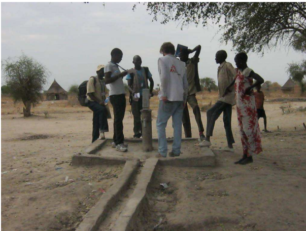
Image 3: The technical team assessing one of the broken borehole
