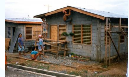
Ph. 3 - Dwellings featuring mixed structure are typical of small towns and urban areas and house the middle class
