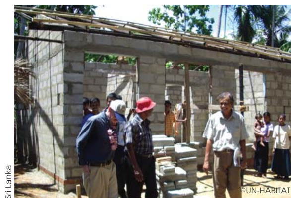
Improving Construction Methods
