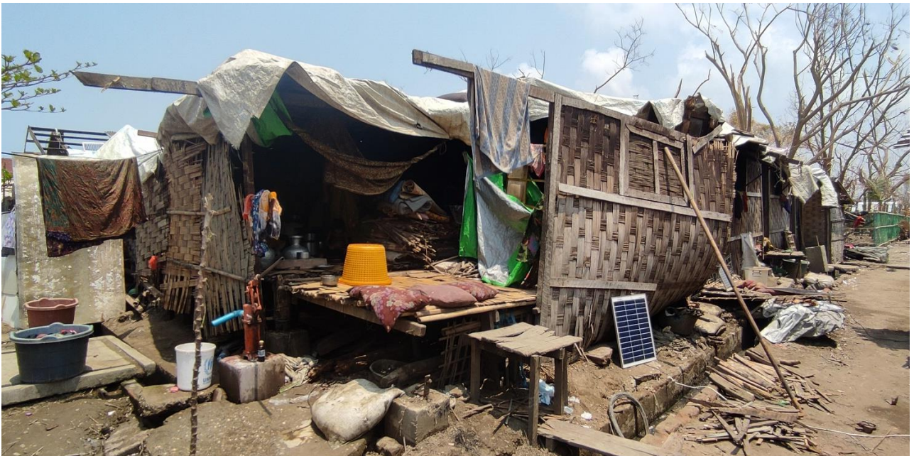
Shelter from Maw Thae Ngar IDP camp – Sittwe township after Mocha cyclone: Some families dismantled their own rooms and set up makeshift shelters as the conditions inside the longhouse were not any more conducive for safe life.
