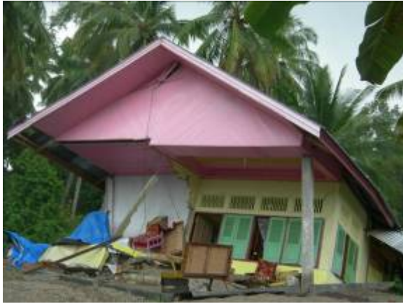
Land movement, causing sedimentation to the foundations, relocation and tenure issues may become important.
