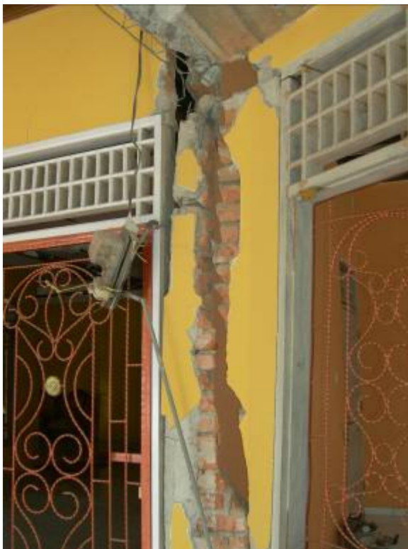
Size of structural columns too small and low quality of re-enforcement bars.
