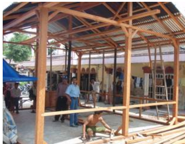
Community start constructing
