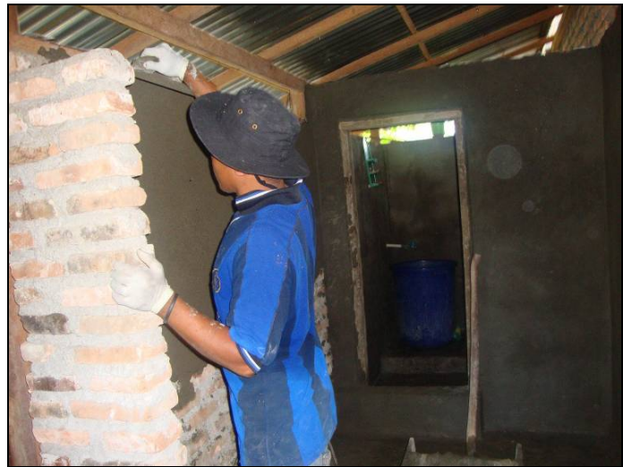
Photo: First stages of construction
