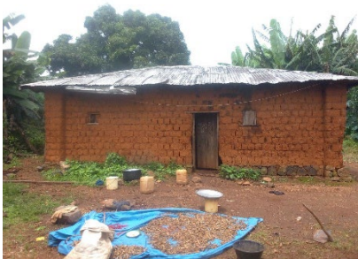
Living inside the house
