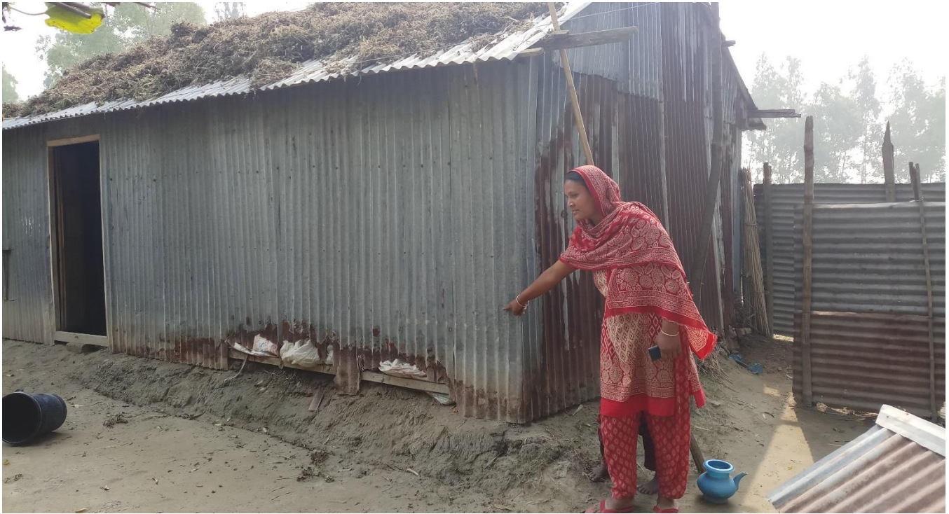
One of the community members marked the flood last flood level, as well as we can see the shelter conditions after the flood.
