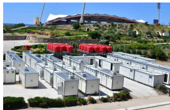
IOM/Al-Rokhsy. IOM rehabilitated shelter at Sport City in Lattakia
