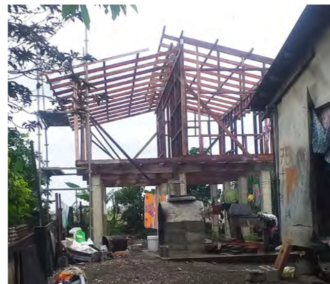
Figure 53: (Below) Hipped roof using timber for framing, galvanized steel strappings and cross bracing.
