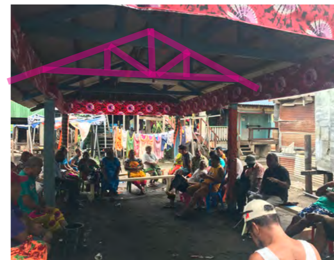
Figure 49: Gable Roof truss with bracing. Location: Ontong Java settlement (Photo credit: John Clemo)
