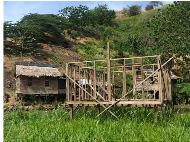
Figure 24: Incremental addition of floor and wall frames. Location: Jabros settlement (Photo credit: John Clemo)
