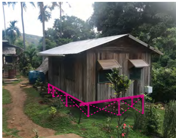
Figure 14: Photo of a typical timber house with timber posts, corrugated roof and window shields for rain; dotted line shows improvement opportunities. Location: Aekafo-Feraladoa settlement (Photo credit: John Clemo)
