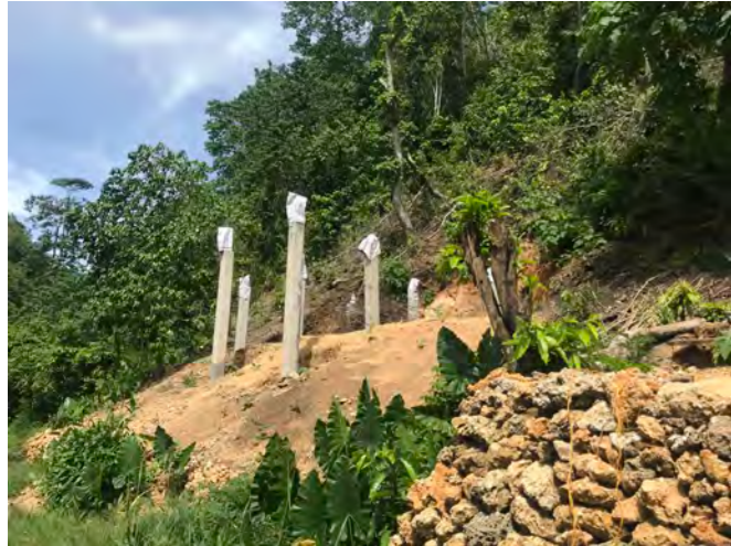
Figure 23: Only footings and posts constructed. Location: Jabros settlement (Photo credit: John Clemo)
