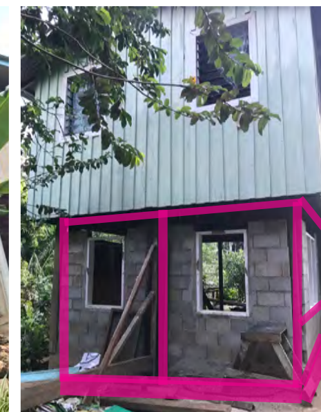
Figure 40: Photo of a house with reinforced concrete strip footing, timber posts, masonry walls and Colourbond roof. Location: Aekafo-Feraladoa settlement (Photo credit: John Clemo)
