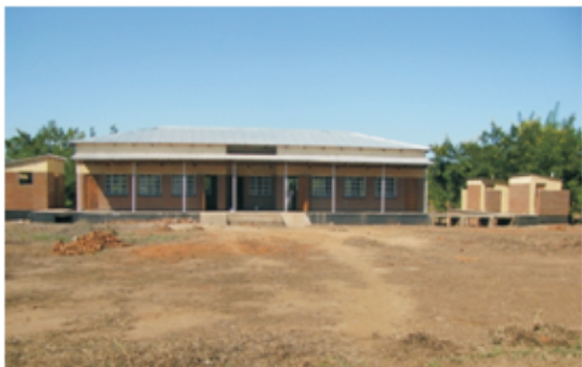
Photo 7 The safe haven complete with toilets and kitchen.
