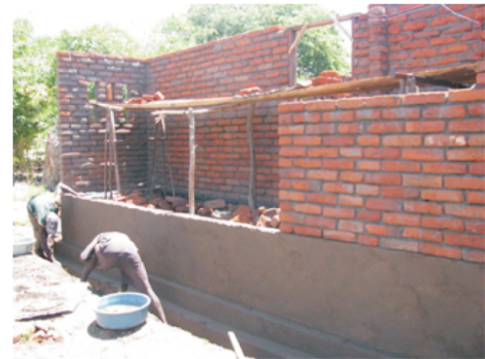
Photo 4 Good foundation construction is the basis of a sound house
