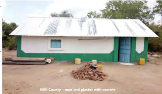
Kilifi County – mud and plaster with cement
