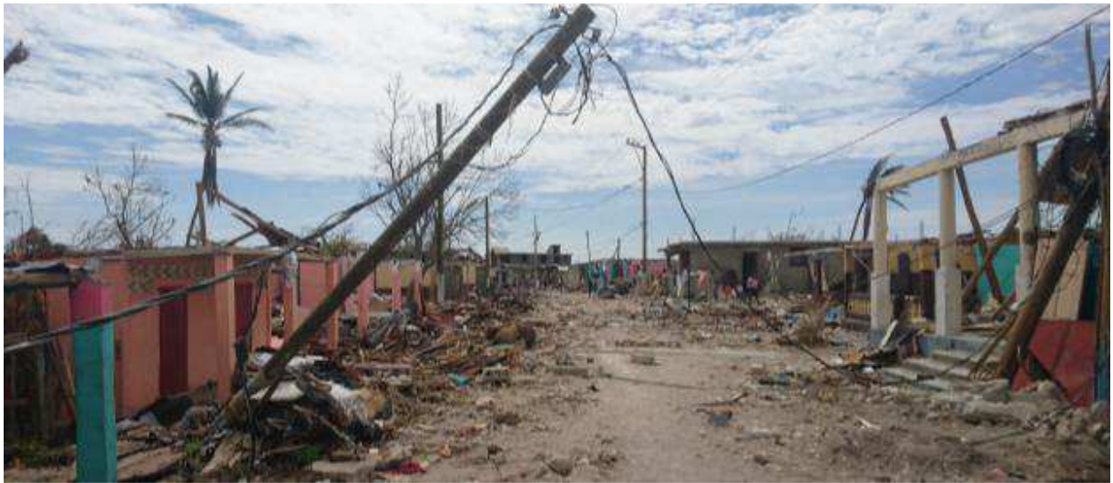
Heavy infrastructure damages
