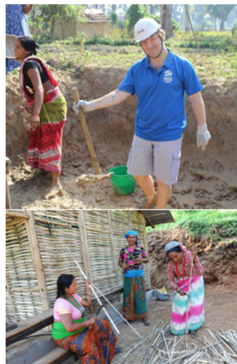
(Top) Working with the local community was an amazing experience for Australian volunteer Richard Riddell. (Bottom) Nepali women cutting bamboo into strips for weaving into wall panels. Photos: HFH Nepal; Mikel Flamm/Habitat for Humanity.
