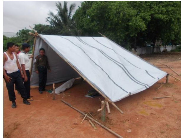
Low single elevated shelter. Good use of dowel to attach roof frame to support posts
