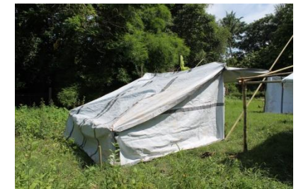
Final roof tarp in place
