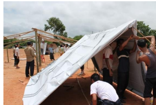
Attaching tarpaulin to frame with bamboo strips
