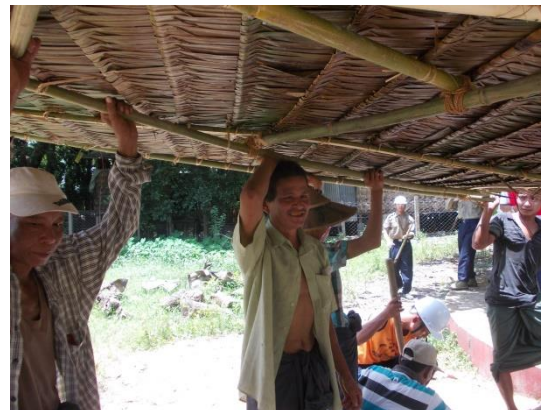
Holding thatched roof up while support posts positioned
