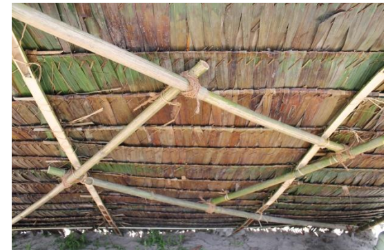
2 split bamboo supports lashed to frame
