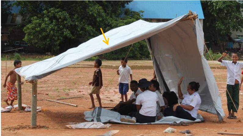
Shelter, the night before rains. Note the single tarpaulin tie (arrowed)
