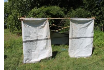
Both side walls completed
