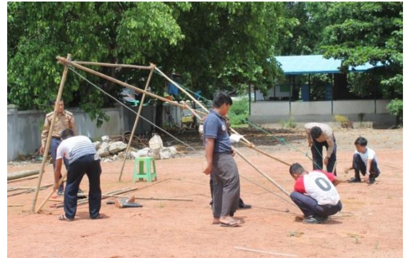
Rope attachment as frame nears completion
