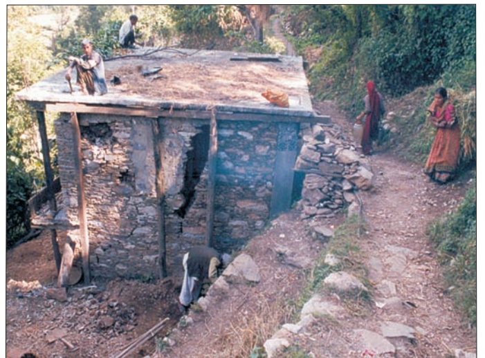
Restoration of stone house in Uttarakhand
