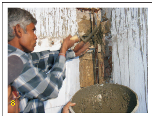
8. Clean all the shear connector holes and fill them up with non-shrink cement cum polymer grout. Making sure that bar is fully encased.
