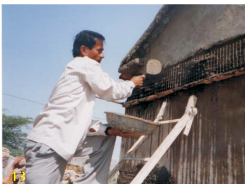
13. Splash the exposed wall surface with water and apply neat cement slurry followed by first coat of cement : sand (1:3) plaster.
