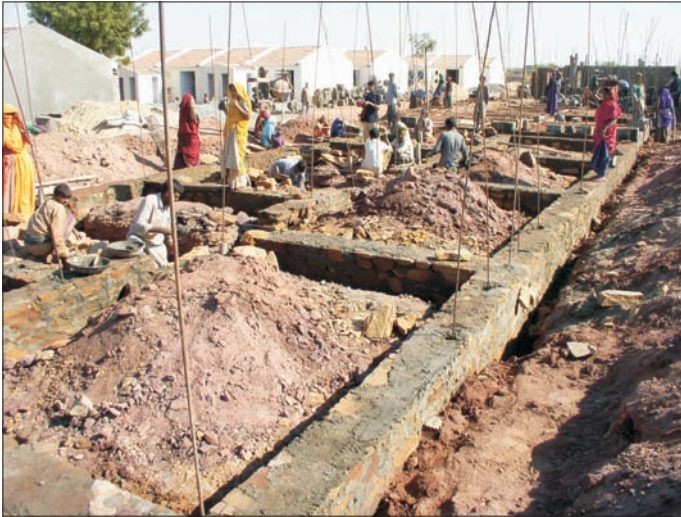
Vertical Reinforcements at all the corners
