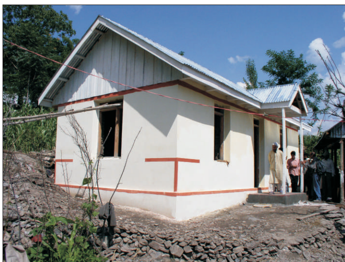
A stone/mud house with GI roof in Kashmir
