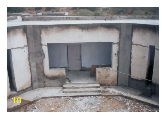
10. Splash the exposed wall surface with water. While still wet, apply neat cement slurry followed by first coat of cement-sand (1:3) plaster of 12mm (1/2") thickness.
