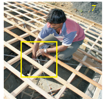
7. Pre-tension wires by twisting all wires along one diagonal together with a piece of rebar.
