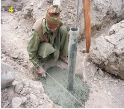
Insert 100mm (4") diameter PVC pipe 900mm (36") long over all vertical reinforcement bars.
