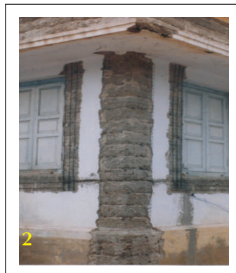
2. Remove the plaster from the marked area and expose the walling material.
