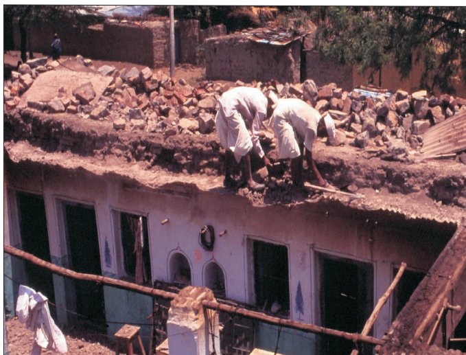
Restoration of flat mud roof in Latur
