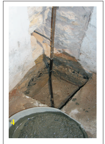
4. Remove 300 x 300mm patch of flooring and excavate to 450mm depth. In the excavation place a bar with bottom 230mm (9") bent in 'L' shape. The rod will pass through each intermediate floor.
