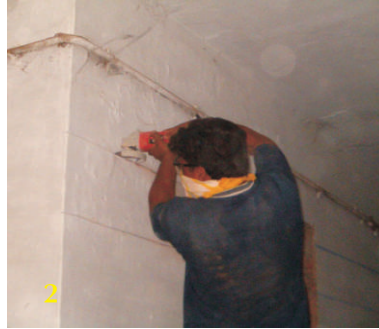
2. Using electric grinder, or chisel, cut the plaster along the markings.
