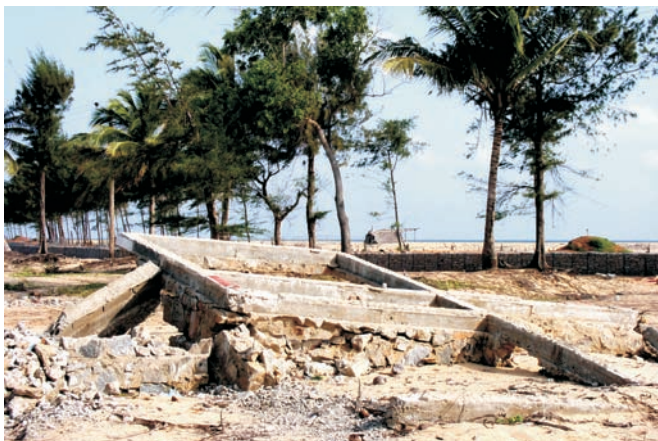
Damage by Cyclonic Surge
