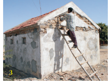
3. Remove the plaster from the marked area exposing wall surface.
