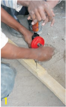
1. Pre-drill planks and rafter /purlins.
