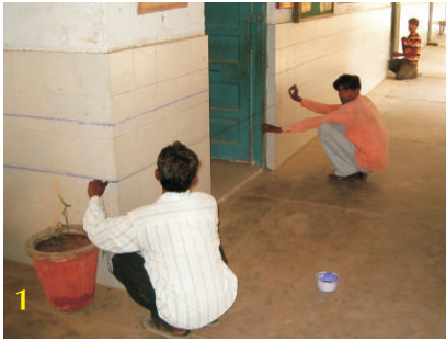
1. Mark the top & bottom edges of belt on wall using string and tube level.
