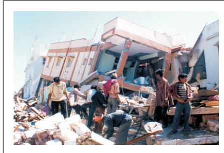
Collapse in earthquake
