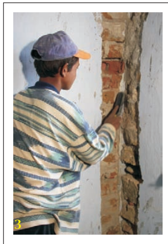
3. Clean the surface with wire brush.
