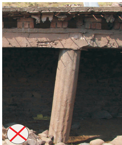
Never do concreting without proper and continuous rodding, or use vibrator
