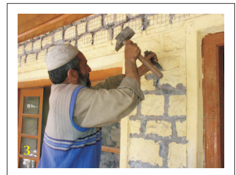
3. Rake all the mortar joints to the depth of 12mm (1/2") by chisel or electric grinder. Clean the surface with wire brush.
