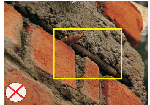
Never place reinforcing bars without or with little concrete cover. They add very little to the strength.
