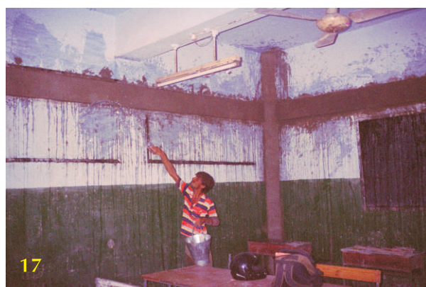
17. Cure the plaster for 15 days.
