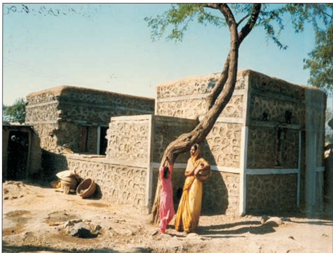
A stone/mud house with flat mud roof in Latur
