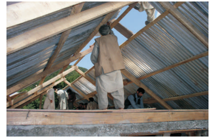
Large Purlins from Truss to Truss
