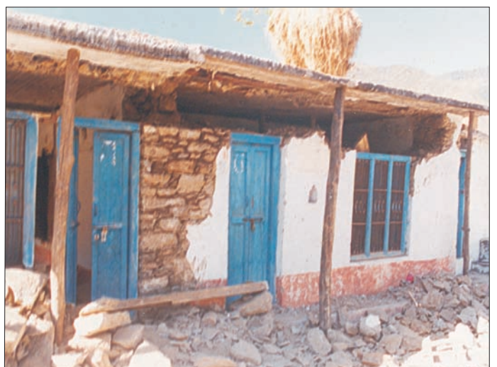
Restoration of stone walls in Uttarakhand
