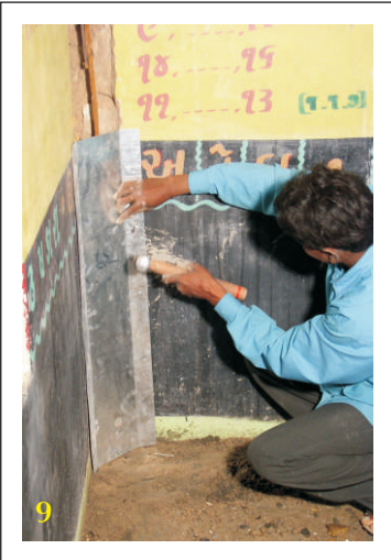
9. Once all the shear connectors are grouted, clean the wall with wire brush and water. Install GI sheet/timber plank centering.
