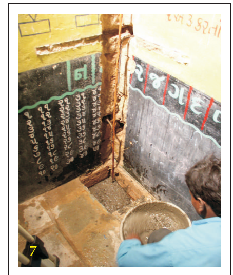
7. Keeping vertical bar in plumb, pour the 1:2:4 concrete with continuous rodding in the hole in the ground to completely encase the bottom of steel rod in concrete.
