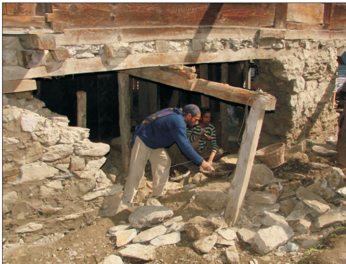
Restoration of a stone/mud/timber house in Kashmir
