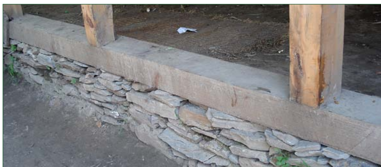
A good plinth protects the base plate and ensures it dries quickly.
