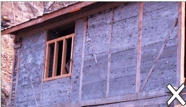
In situ concrete infill.
