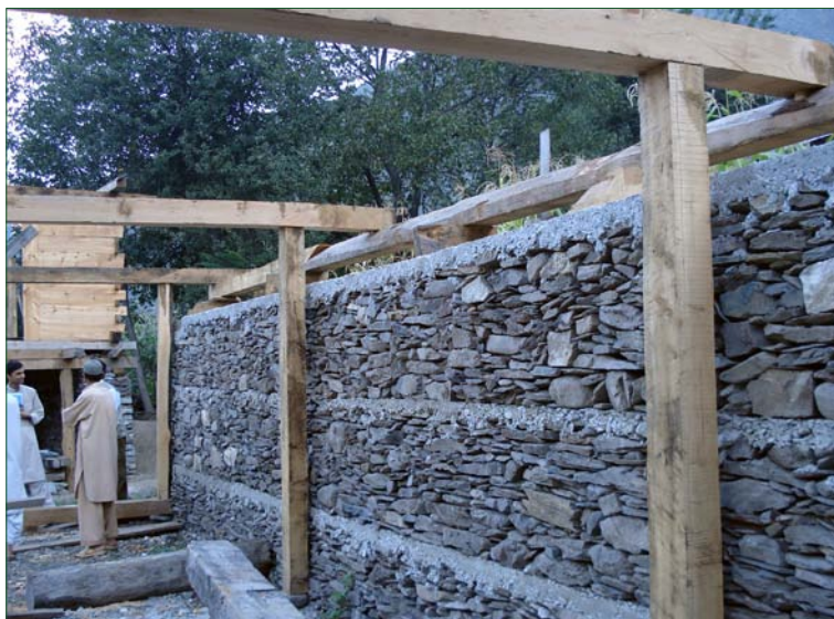
Timber posts inside and separate to the wall. RCC bands between well laid dry stone masonry.
