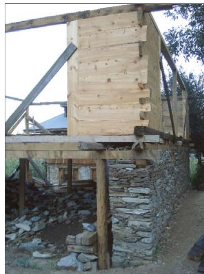
Upper storey frame is fixed to top of the wall.
