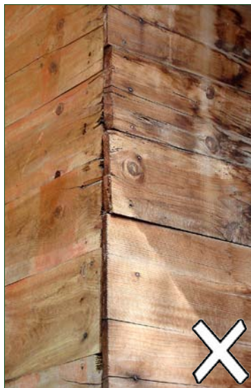
Thin boards may split or warp, nailed at weak location.
