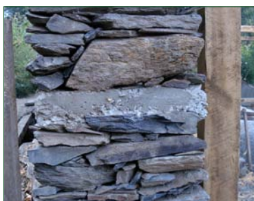
RCC bands can strengthen the wall.
