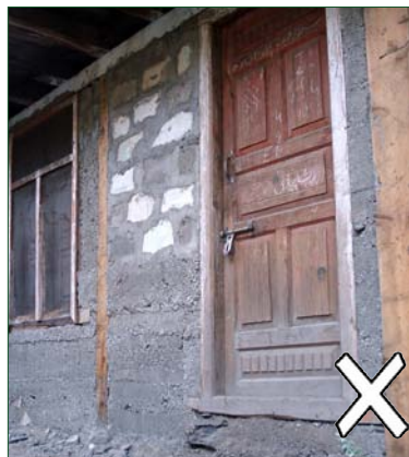
Masonry with sand cement mortar.
