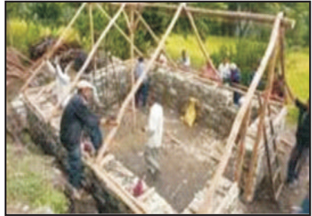
Four sets of rafters installed on ridge beam.
