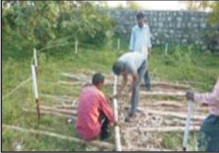
Prepare timber ballis for wall plate
