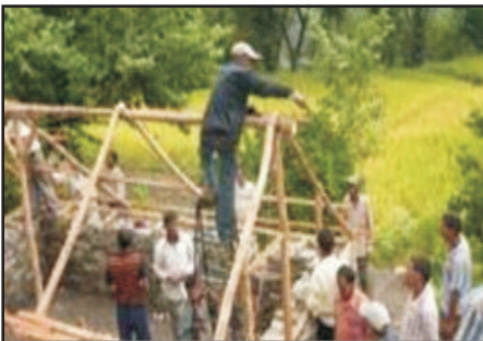
Install 4 purlins on each side of the roof with nails. Using spirit level or tube level ensure that all the purlins (batons) are level (not sloped).
