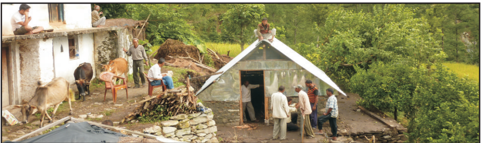
Step by Step Construction of a Semi-Permanent House - NCPDP
