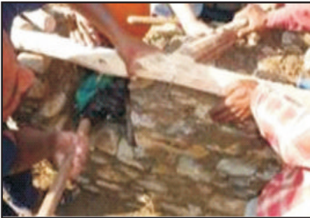
Attach 12" to 13" long ( flush with the inside face of the wall) ballis stiffeners with metal straps and nails.
