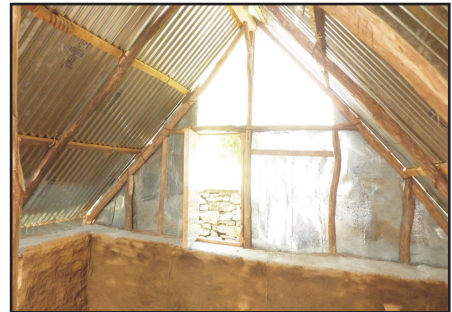
Windows in the back wall which gives extra light and ventilation. The top hung shutter acts like a chajja.
