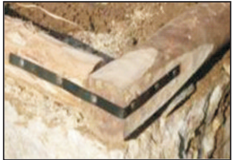
Timber to timber metal strap connector.
