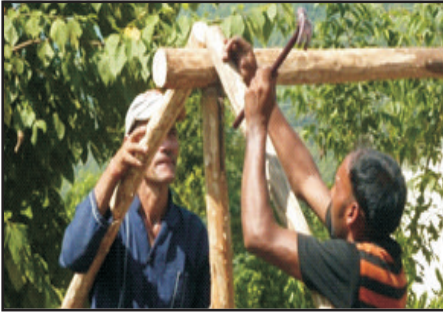
Rafter and ridge beam connection
