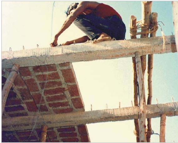
Pre-cast bk. panels supported on pre-cast RC joists
