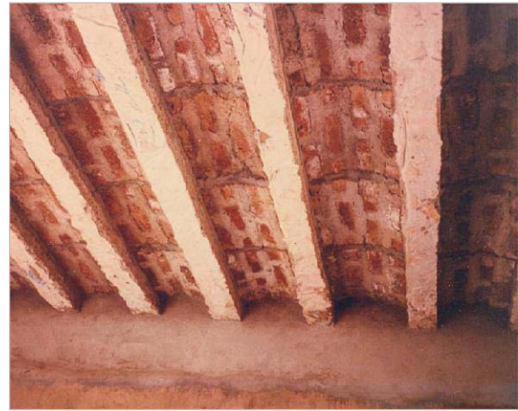
Burnt brick Jack Arch supported on RC joists.
