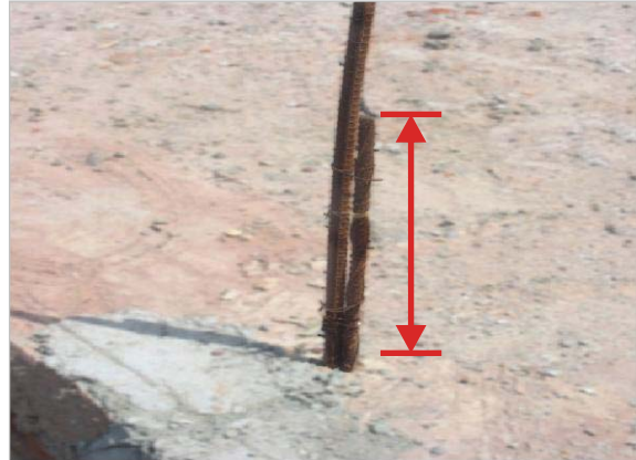
All bars must have proper overlapping joint of minimum 20" (500mm).
