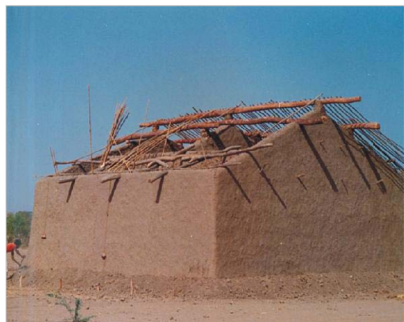
Hand moulded cast in situ mud wall or Cob wall
