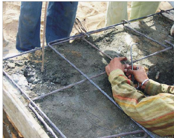
All bars must have proper overlapping joint of minimum 20" (500mm).
