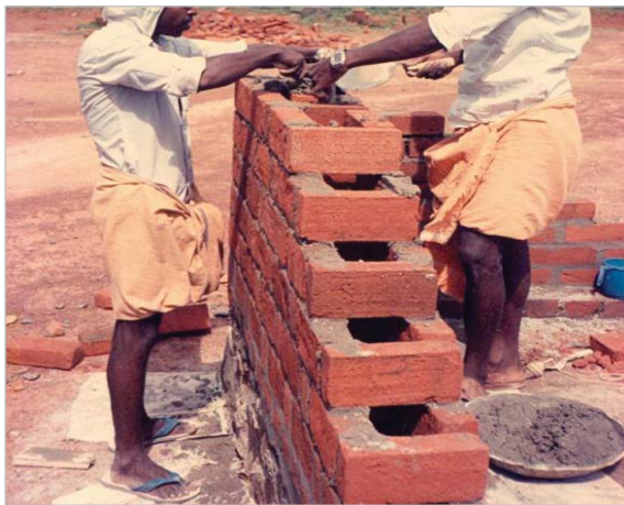
Rat-Trap bond 9" cavity wall.
