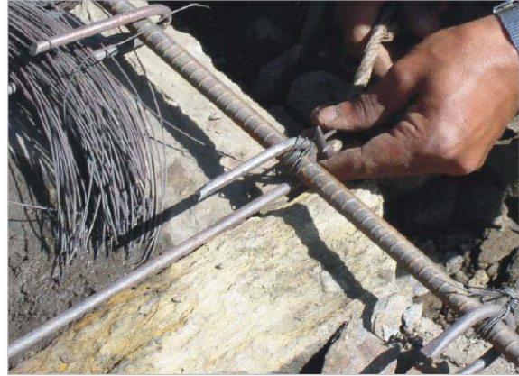
Bar-to-bar connection can be hooked only in cross-links in the RC band.
