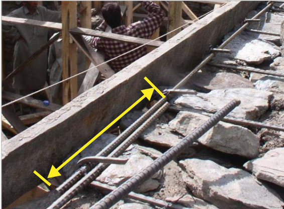
All bars must have proper overlapping joint of minimum 20" (500mm).
