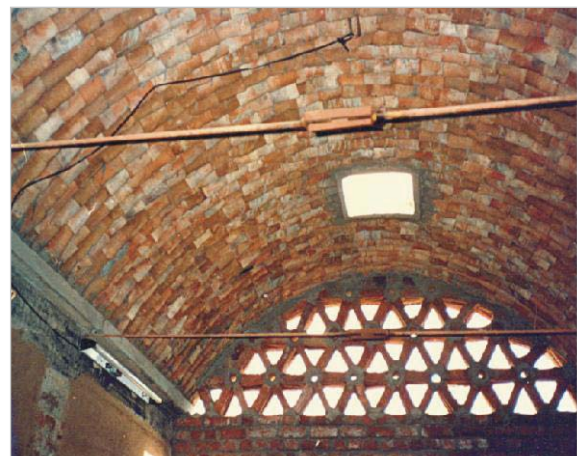
Burnt clay tubes (BCT) vault.
