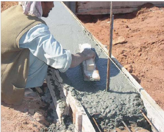
All bars must have proper overlapping joint of minimum 20" (500mm).
