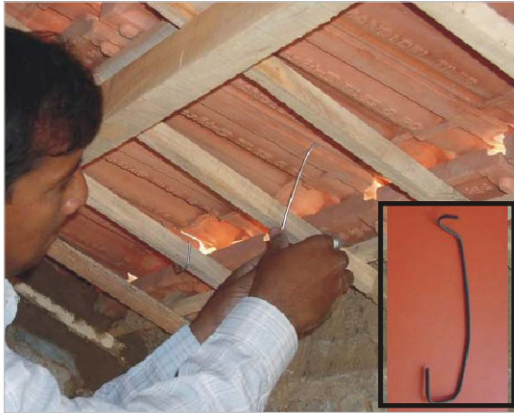
All tiles must be anchored to rafters with GI wire hooks.
