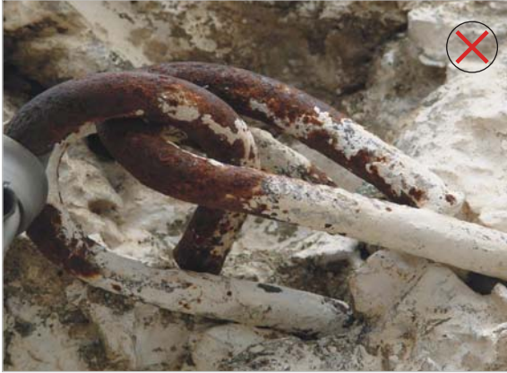
Connection of one bar to other must never be with hooks.
