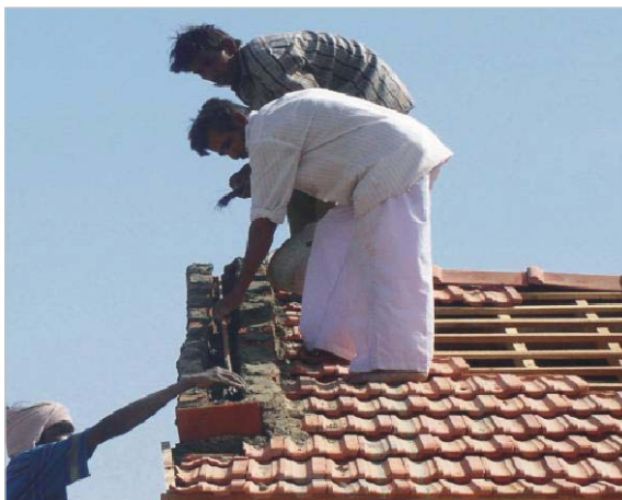
Keep gable top load wall no higher than 9''(230 mm), and reinforce it with a rebar.
