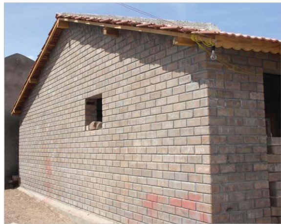
Compressed stabilised soil blocks in Soil-Cement mortar or Compressed Soil Blocks in ordinary mud mortar.
