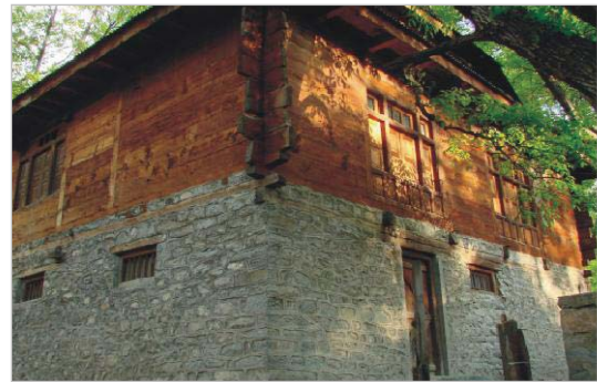
Or with the lower storey in stone, the top storey can be in timber or tin.
