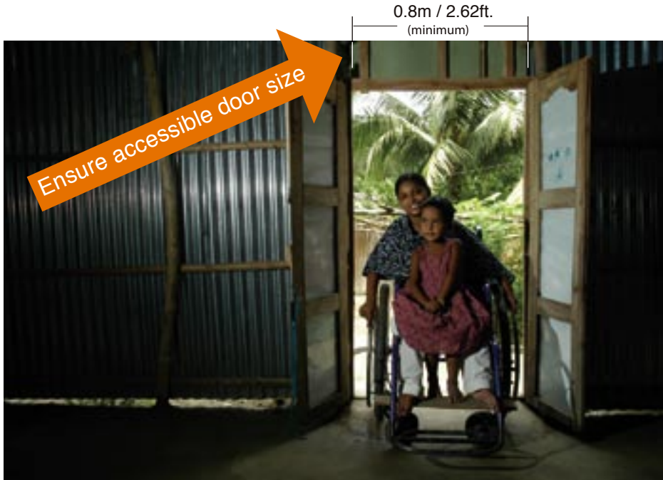
Accessible house with proper door size
