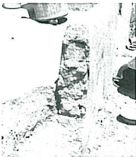
This foundation wall was made from unstabilised earth blocks which have started to collapse
