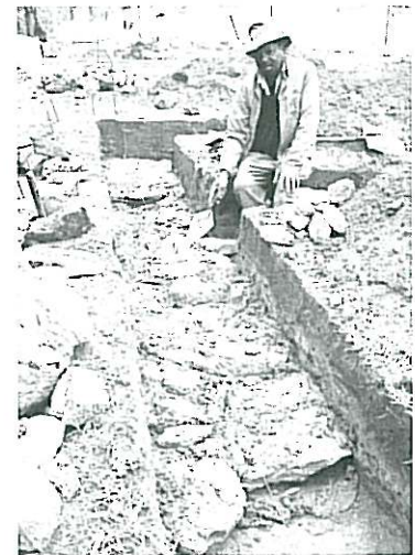
Local stone can be used to make foundations
