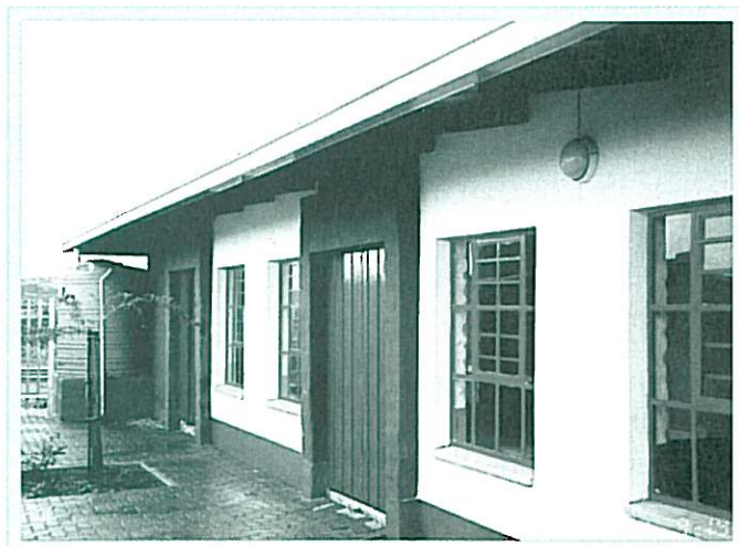
The housing support centre at Waterloo, KwaZulu-Natal, built with stabilised earth blocks
