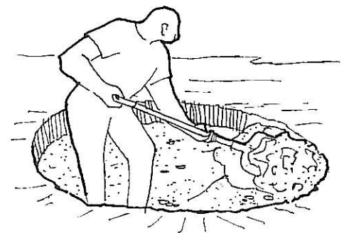
Mixing soil in a pit
