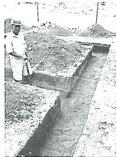
Making trenches for the foundations
