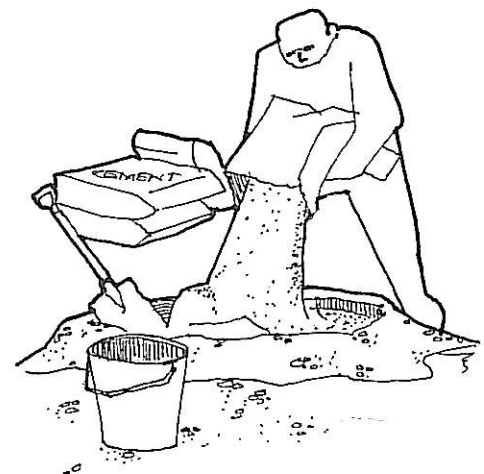
Mixing dry soil with cement to make stabilised blocks
