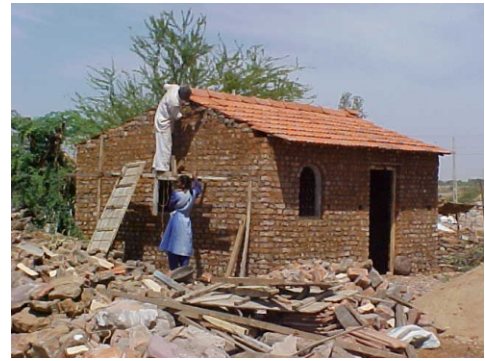
A villager rebuilding his house with unreinforced masonry
