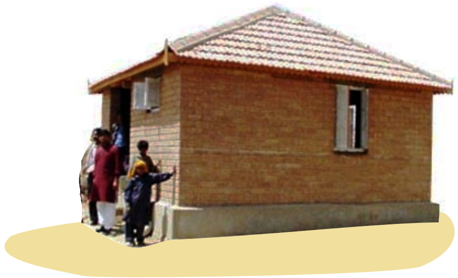
A village house with unreinforced masonry
