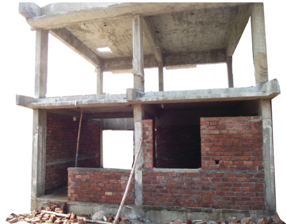
An RC frame building commonly built in cities
