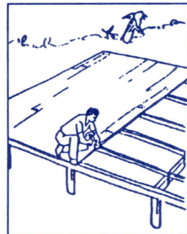
Nail floor boards to joists
