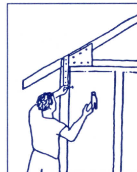
Fasten truss to wall with straps
