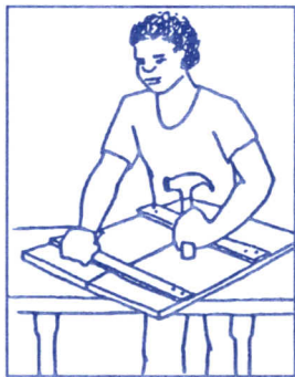
Saw and nail boards to make strong shutters
