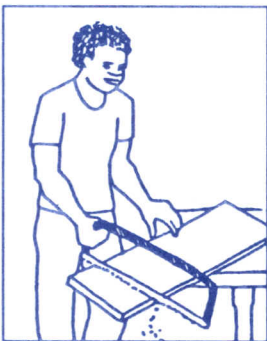
Saw and nail boards to make strong shutters
