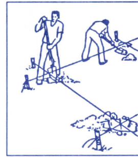
Dig post holes
