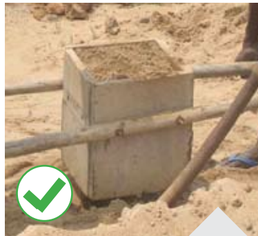
Good system of batching
