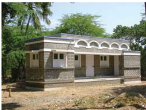
Flyash Brick Masonry Florida Construction-UNDP
