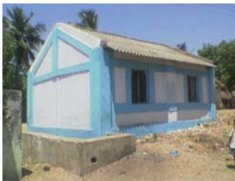
Retrofitting technology demonstration unit by SEP and UNDP
