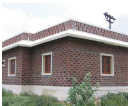
Rat - Trap Masonry COSTFORD and UNDP
