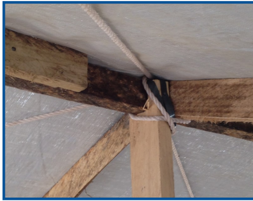
Key joints are improved with metal straps (langa langa) and/or rope.
