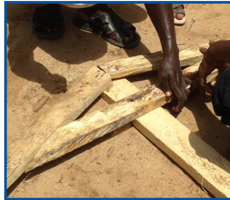
Strengthen the truss by adding bracing
