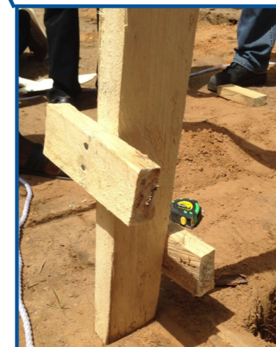
Anchor the foundation...
