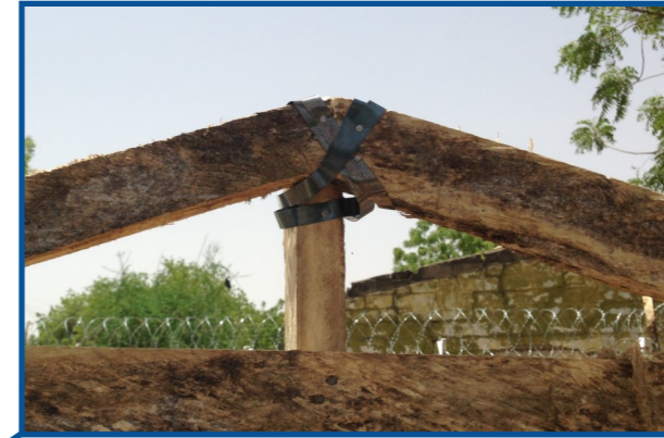
Langa langa to strengthen key joints.
