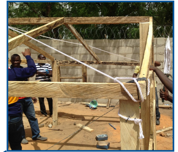
Roof bracing can be done with rope.
