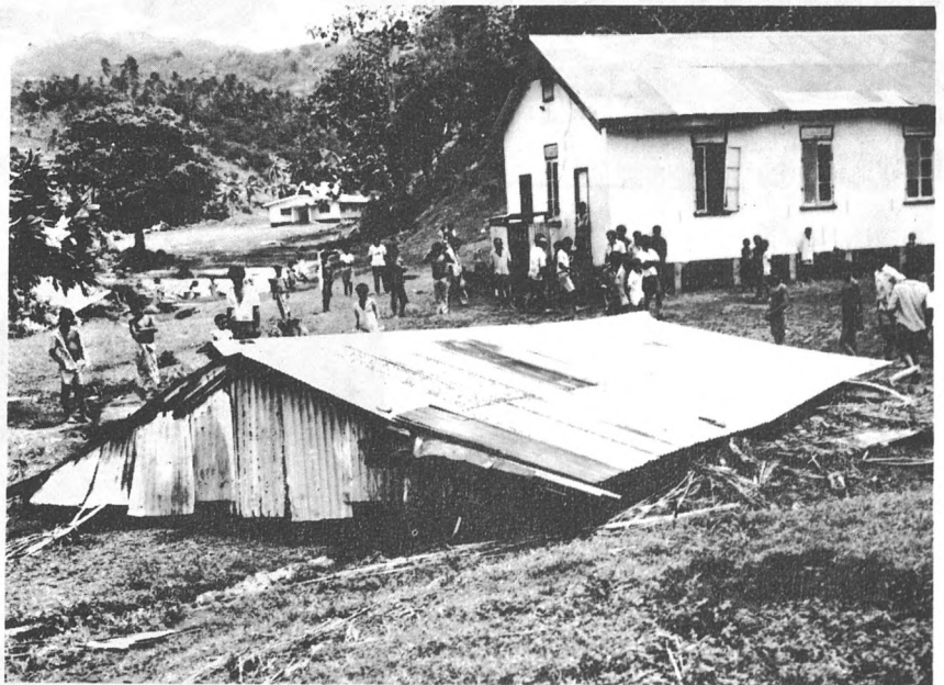
Inadequate Fastenings of Roof to Walls
