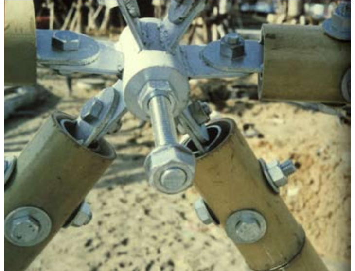
Bamboo connection in metal by Shoei Yoh 1
