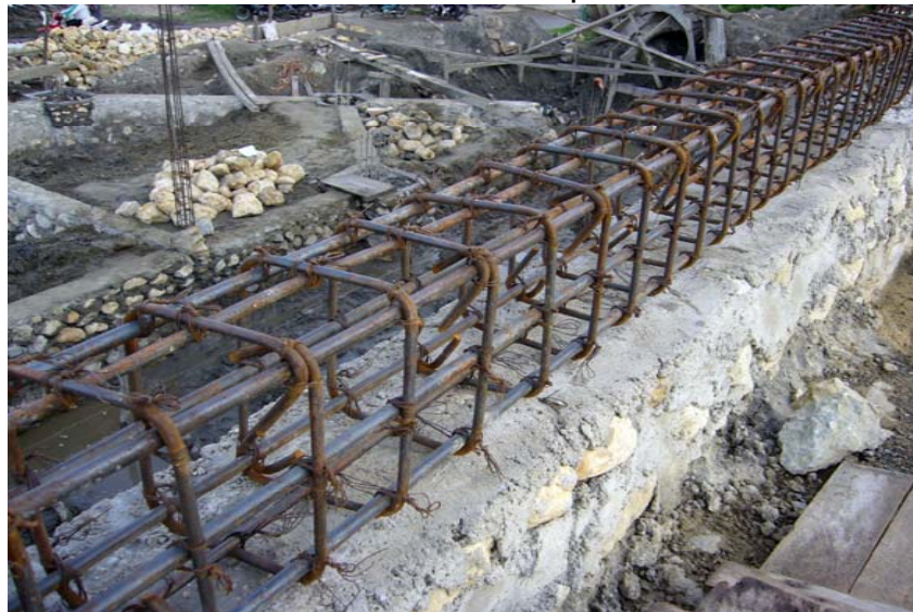
Ends of steel bent at 135° for earthquake resistance.
