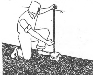
Correcting the level of the finished floor Rectificando el nivel de piso acabado
