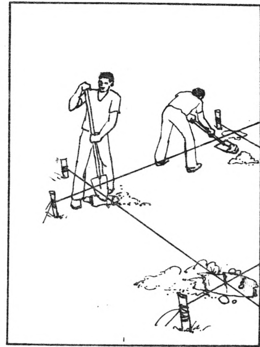
DIG POST HOLES
