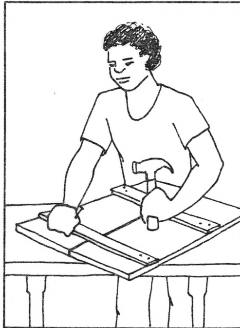
SAW AND NAIL BOARDS TO MAKE STRONG SHUTTERS
