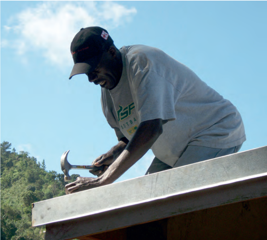
Jamaica: Installation of fascia cap over fascia board. (© French Red Cross)
