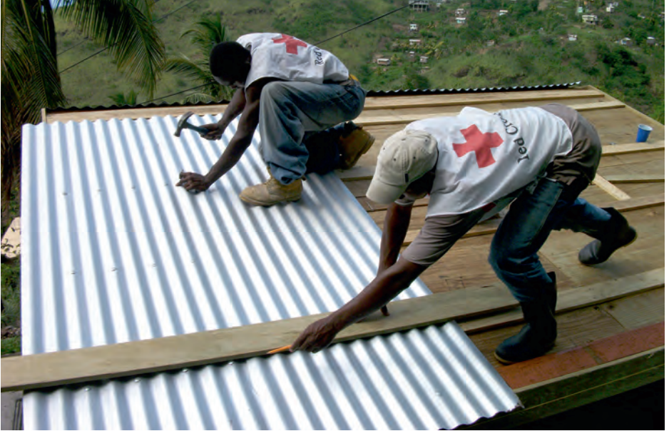
St Vincent & Grenadines, Hurricane Tomas, 2010: Installation of CGI sheets, cord at eaves overhang to line up the CGI sheets, marking of the location of the laths in order to better place the roofing nails. (© French Red Cross)
