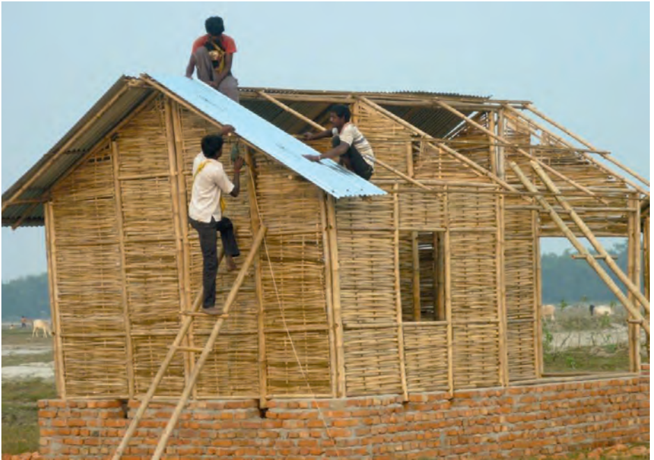
Nepal: Installing CGI on bamboo structure. (IFRC-SRU)
