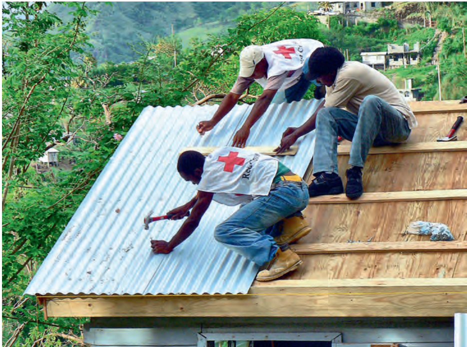
St Vincent & Grenadines, Hurricane Tomas, 2010: RC volunteers installing CGI sheets on a gable roof. (© St Vincent & Grenadines Red Cross)
