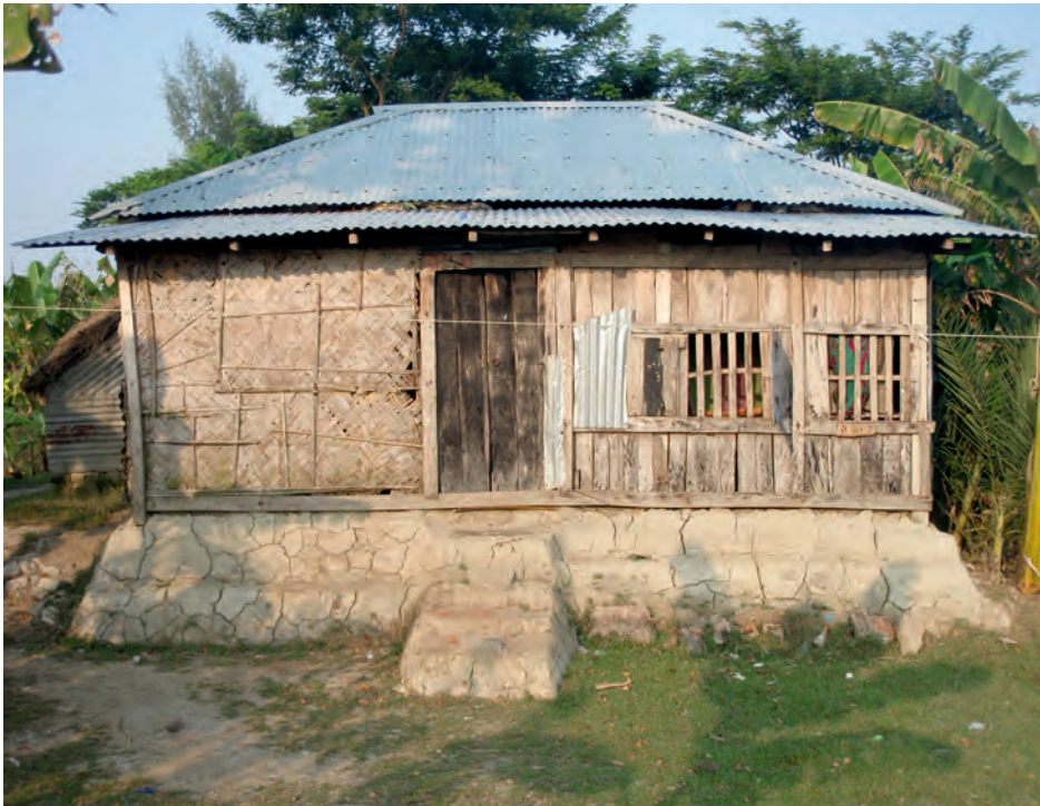
Bangladesh: House with ridge and hip capping. (IFRC-SRU)
