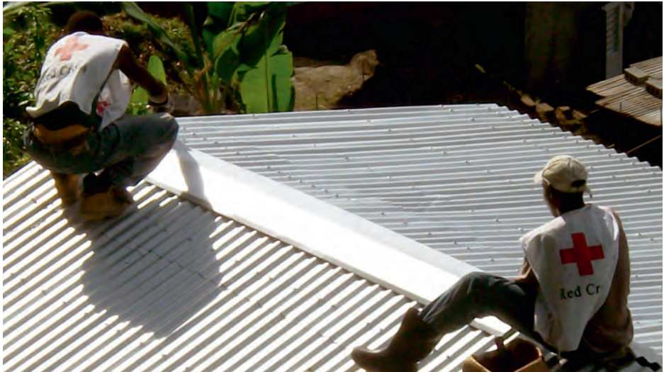
St Vincent & Grenadines, hurricane Tomas, 2010: RC volunteers nailing a ridge cap. (© French Red Cross)
