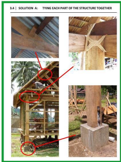
DRR Training – Shelter resilience | M3 - How to increase sturdiness of the building | CRAtene 21
