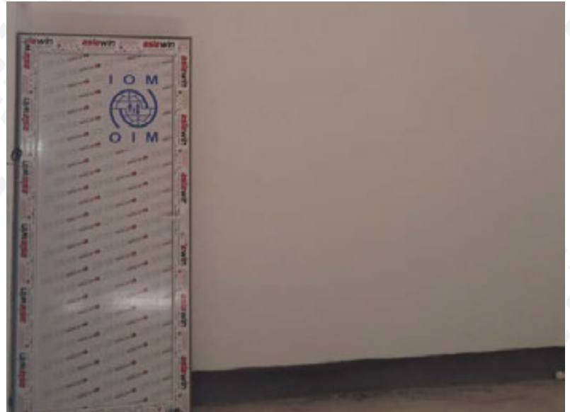
Family room wall rehabilitated with electrical fixtures; painting completed.
