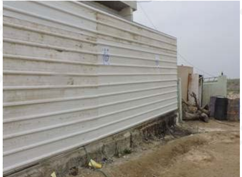
Fenced perimeter offers protection against vulnerabilities such as intrusions.
