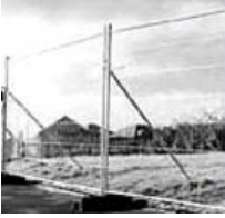
a wire net fence showing a stiffening brace
