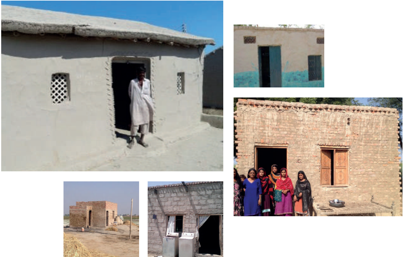
Figure 04. Shelter typologies (clockwise from top): loh kat, adobe, burnt brick, concrete block, burnt brick
