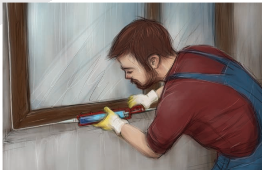
▶ Use the silicone to fill around window frames.
