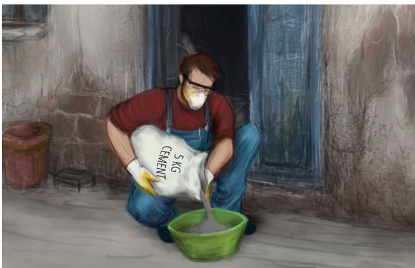
▶ Put 5 kilogram of cement mortar (pre-mixed of cement and sand) in a bucket to cover approximately 2 square meter of surface.
