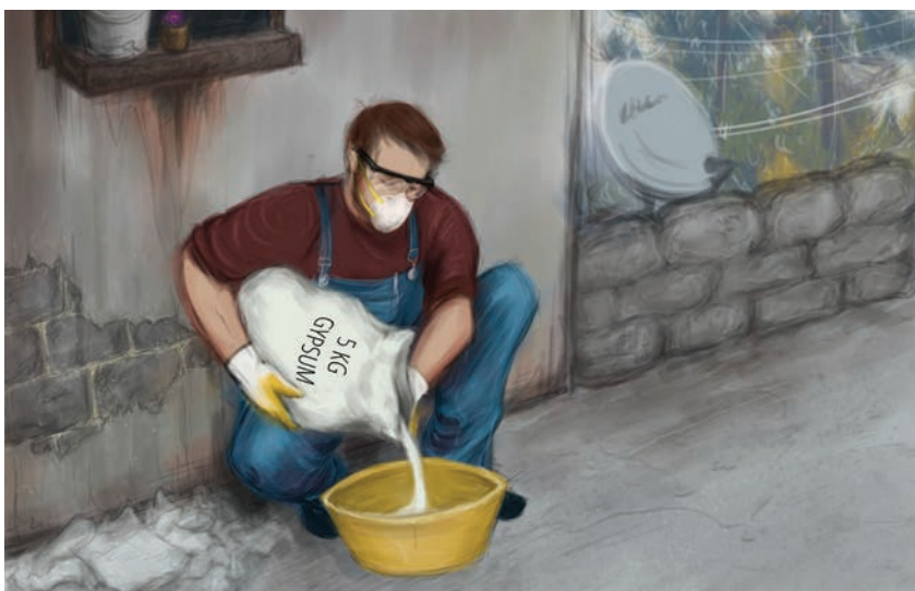
▶ Put 5 kilogram of gypsum in a bucket to cover around 4-5 square meter.
