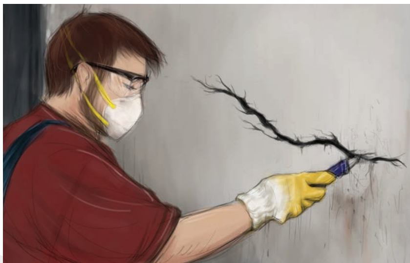
▶ Clean inside/around the cracks using an adjustable knife or scraper.
