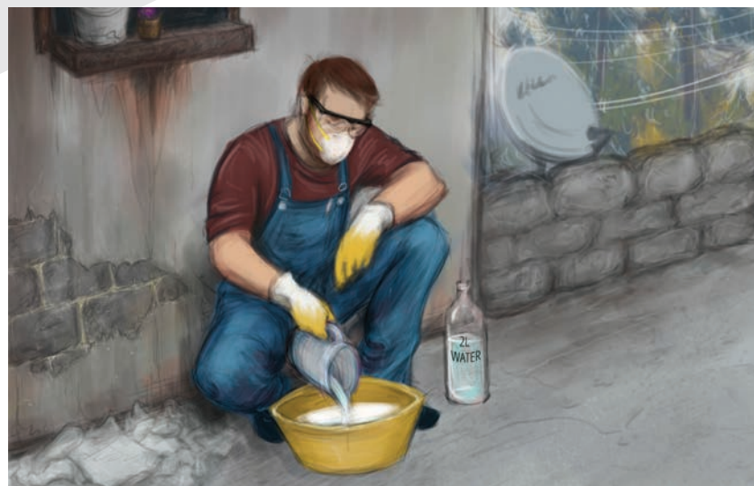
▶ Add 2 liter of water to 5 kilogram of gypsum.
