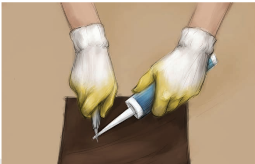
▶ Cut the plastic tube end in a V shape length using a steel knife.
