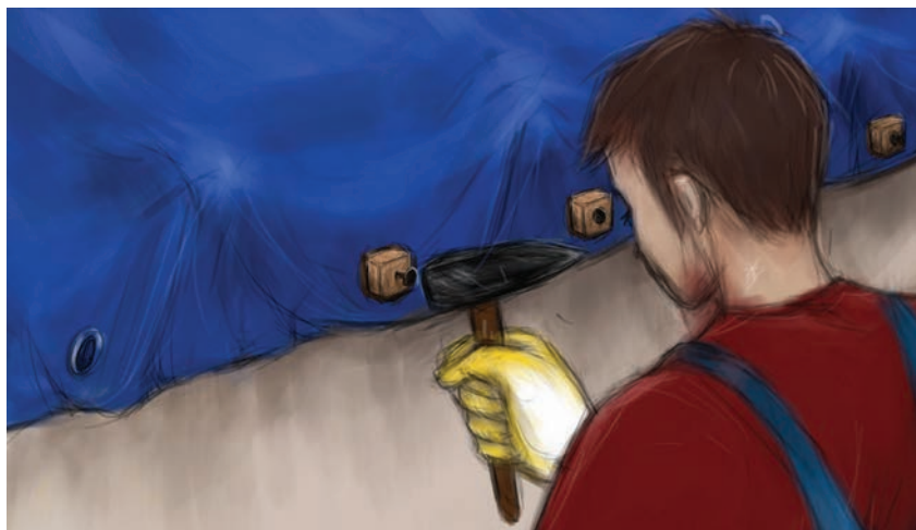
▶ Using timber battening to fix the sheets with iron nails.
