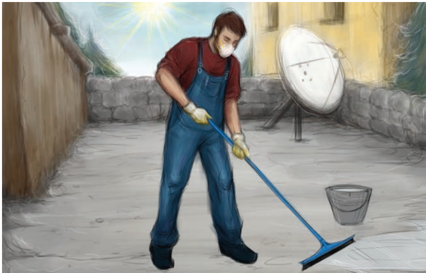
▶ Wash the roof area with water using a rubber sweeper.
