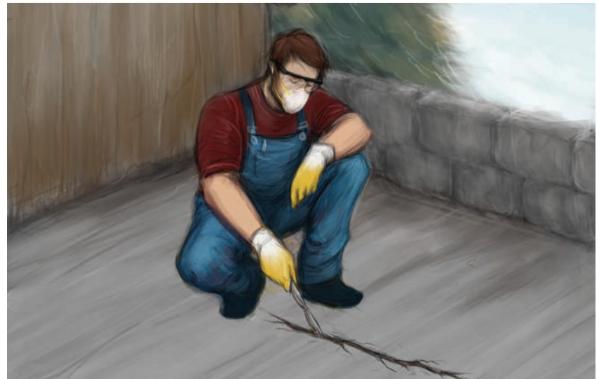
▶ Find any cracks in the roofing and clean them well using a scraper.
