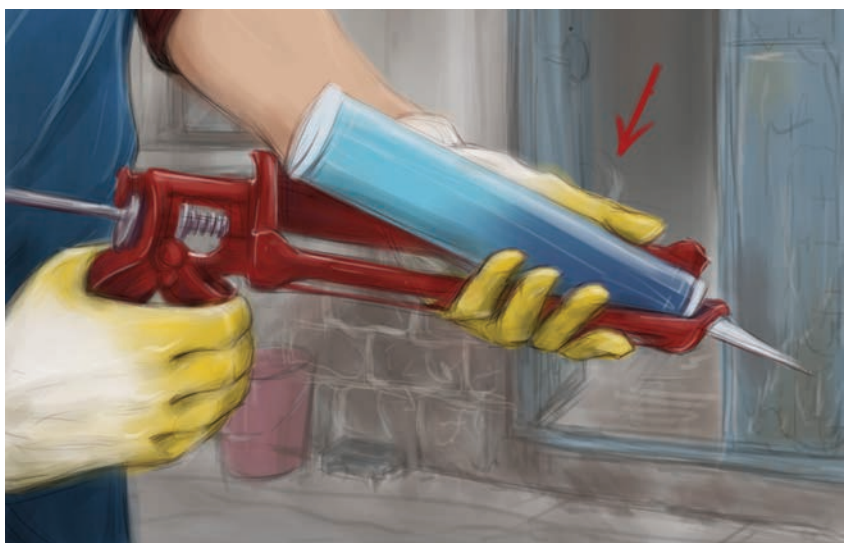
▶ Fill the silicone gun with the waterproof silicone.
