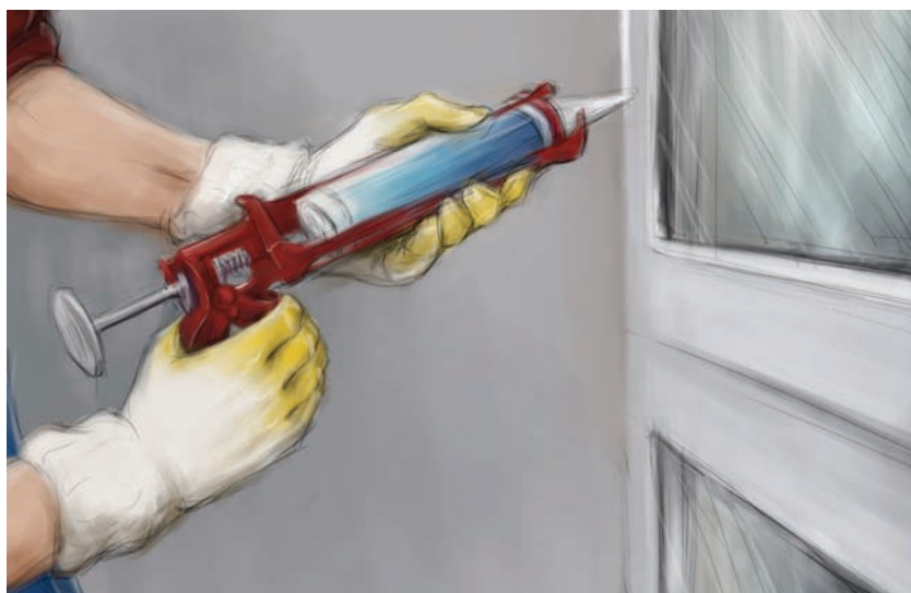
▶ Use the silicone to fill around door frames.
