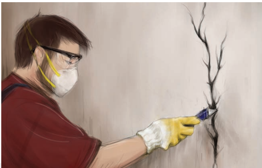
▶ Clean inside/around the cracks in the plaster using an adjustable knife or steel scraper.
