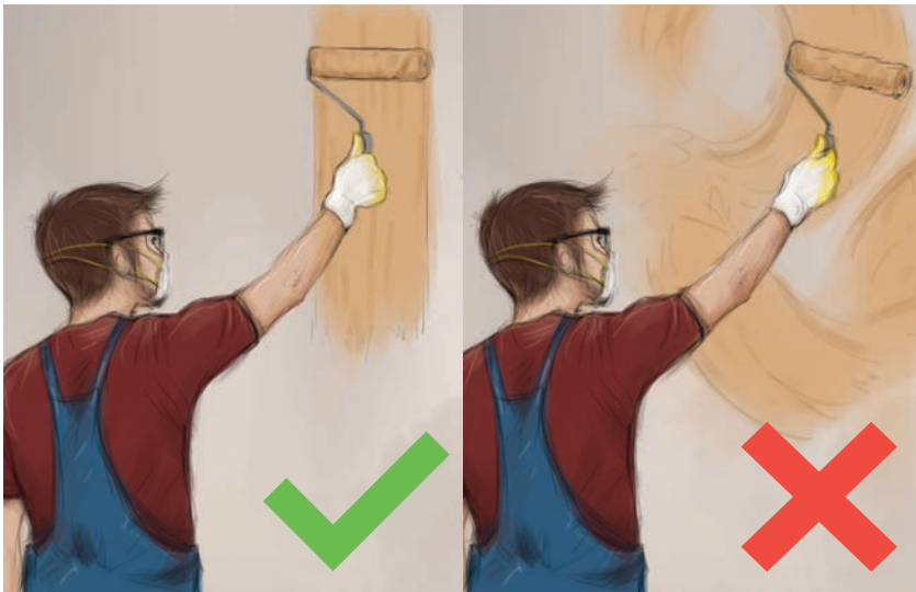
▶ Do not apply paint randomly and use a roller brush for the ceiling and large areas.
