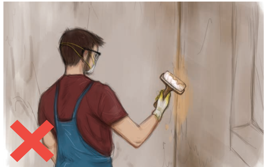
▶ Do not use a roller for corners, be sure to use a brush for these areas.
