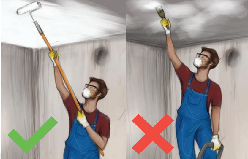
▶ Paint should be applied in one direction only.
