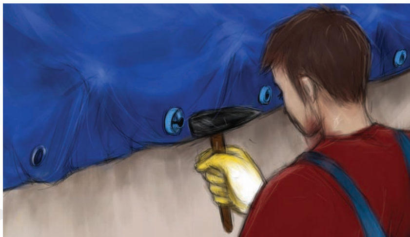
▶ Using washers or bottle caps to fix the sheets with iron nails.
