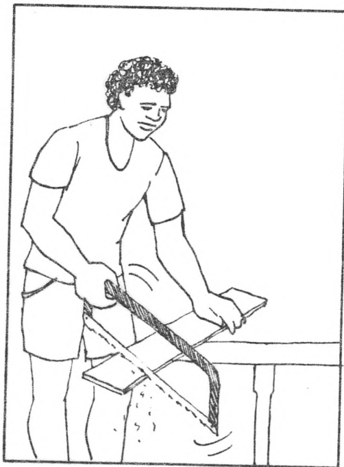
CUT WOOD BRACES
