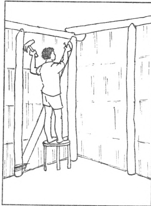
MAKE DIAGONAL BRACES
