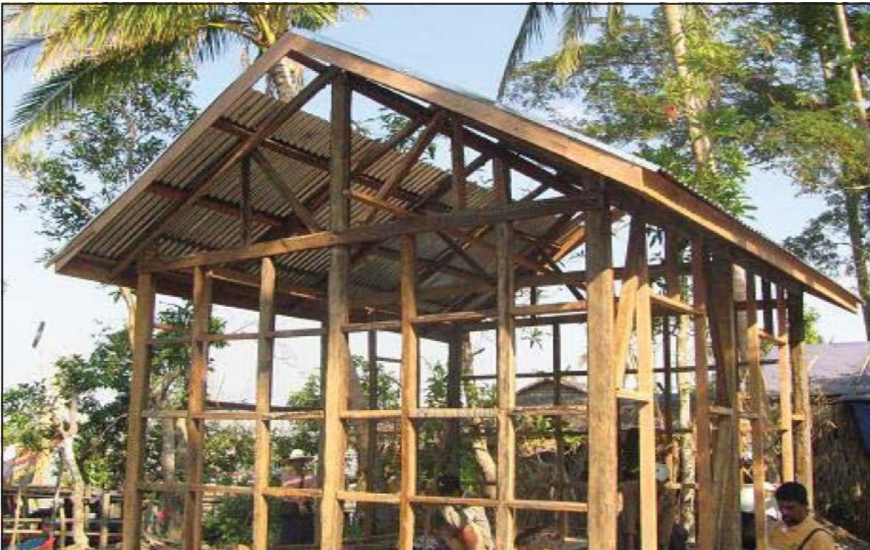
Framework for wall cladding ▲
