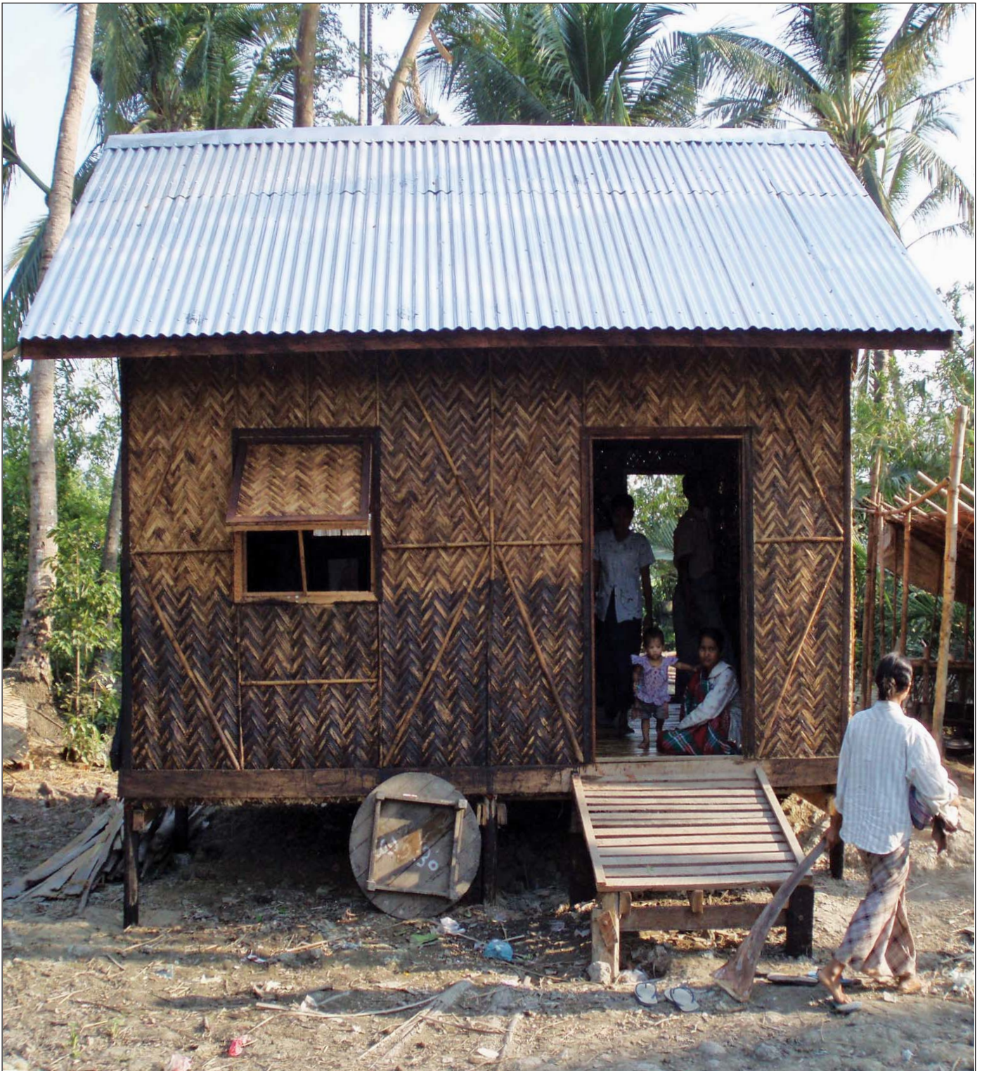
A new shelter complying with DRR requirements
