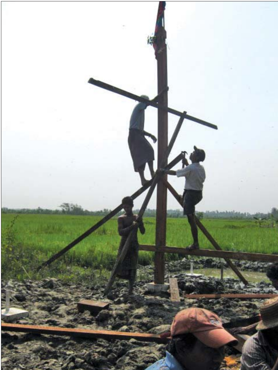
Posts held in position with temporary supports ▲
