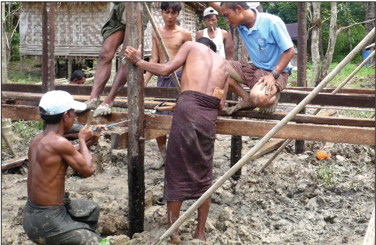
Fixing floor joists ▲
