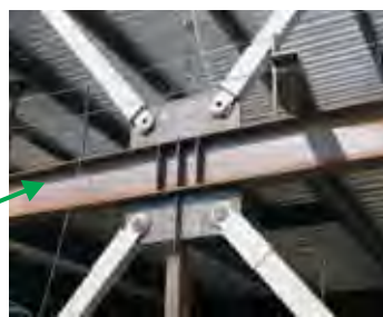
BUCKLING RESTRAINED BRACED FRAME
