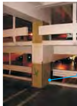
FIBER-WRAPPED SHORT COLUMNS Courtesy Saif Hussain, Coffman Engineers
