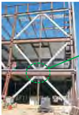
BUCKLING RESTRAINED BRACED FRAME
