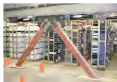
BUCKLING RESTRAINED BRACED FRAME
